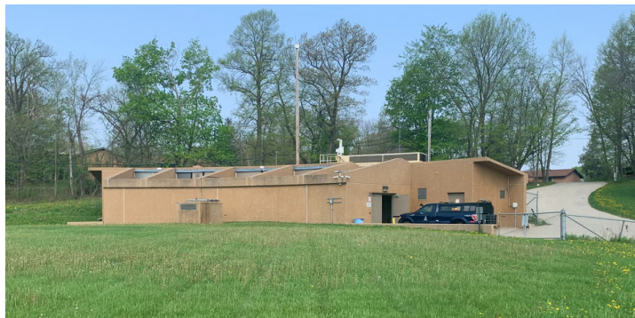
A view looking northwest at the front of the wellhouse and over the buried reservoir. Eagle Heights is behind the tree line across Lake Mendota Drive.
