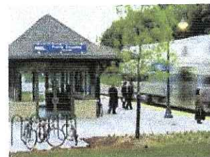
The Prairie Crossing Station
