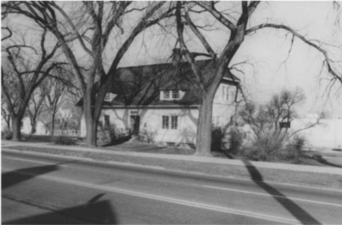
University Avenue frontage
