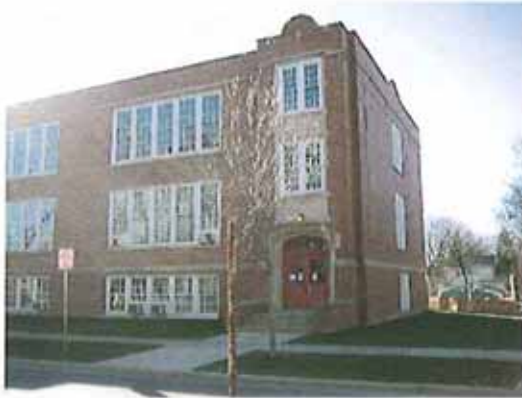
A. 210 S. Brooks St. View looking west on Brooks St.
