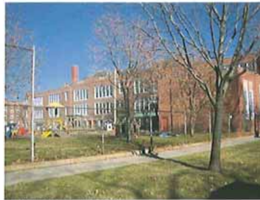
A. 210 S. Brooks St. View looking east on Chandler St.
