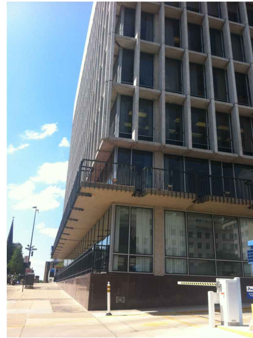
VIEW FROM DOTY STREET
