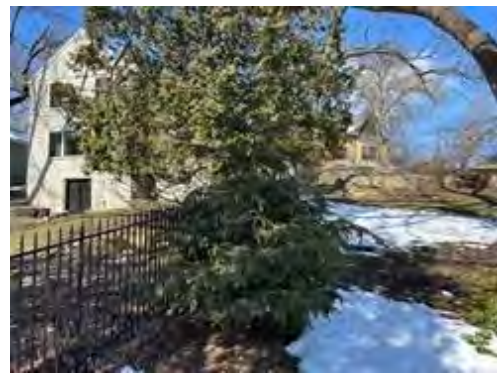
Rear View with Exposed Basement from Back of Our Lot
