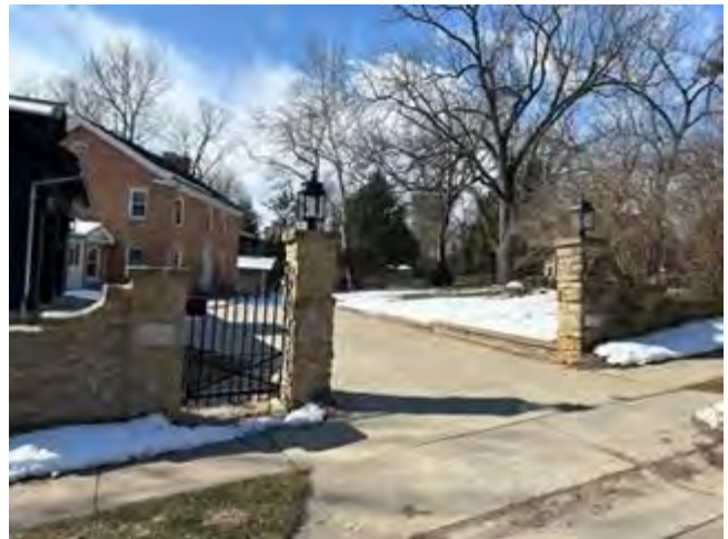
Tavern Driveway, Entrance and Parking Pad off Spring Trail
