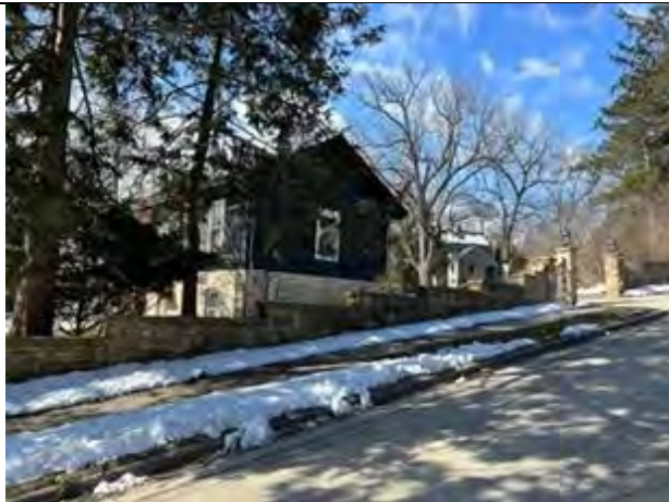
View from Spring Trail of Tavern Garage and Entrance
