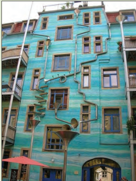
Rain drainage system Dresden, Germany
