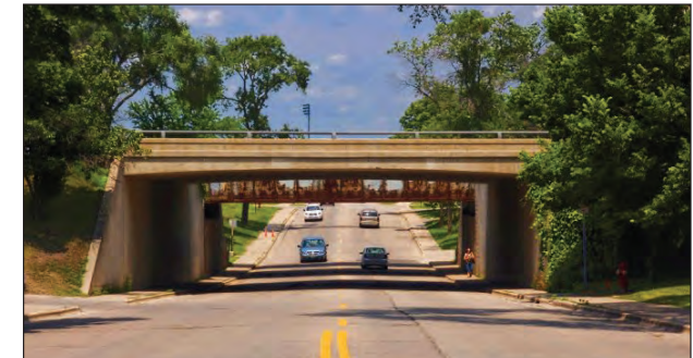
Current view of bridge underpasses
