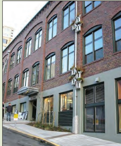
Rain drainage system, Seattle, WA
