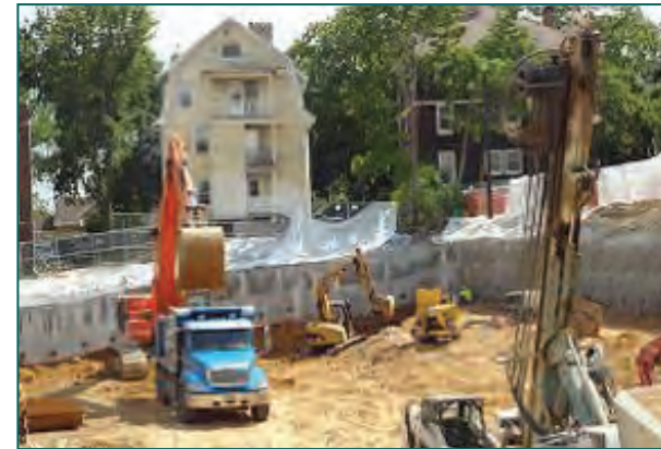
Construction of Brownlofts Apartments, University Avenue, 2013.
