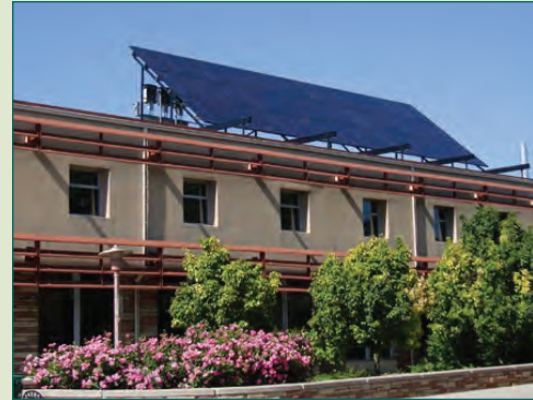
Solar panel example
