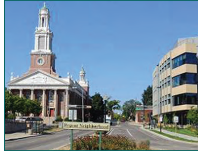
First Congregational Church (left) and Wisconsin Energy Institute (right)
