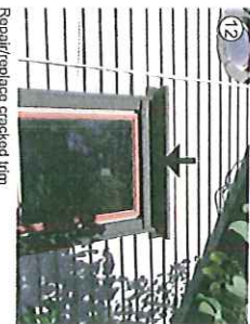
11 Repair/replace cracked trim
