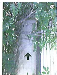
2 Repair cracked foundation
