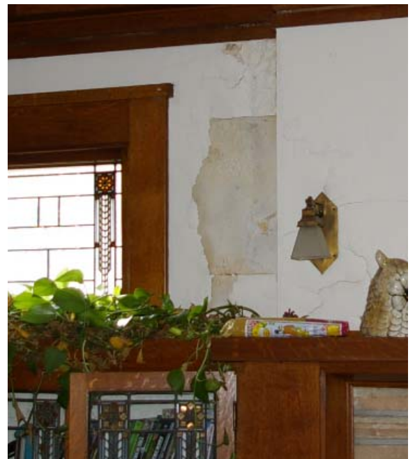
left: condition of the chimney viewed from driveway bottom right: visible interior water damage at the first floor fireplace due to chimney deterioration middle right: condition of the masonry at the northeast corner and downspout draining towards foundation top right: existing unprotected rubber roofing membrane and visible penetration allowing water to deteriorate the wood roof porch structure
