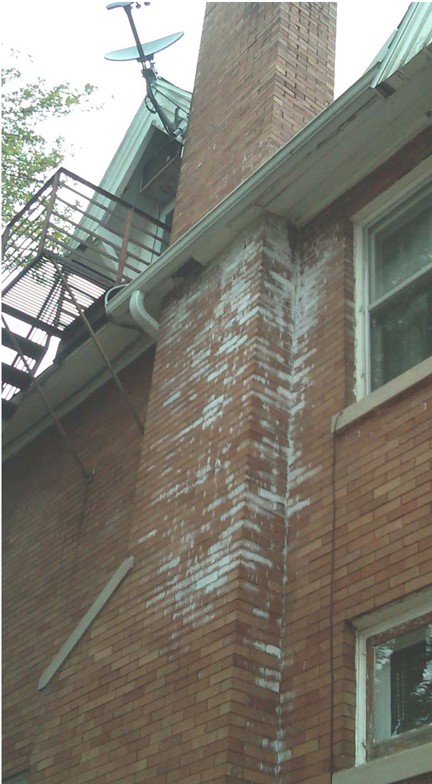
left: condition of the chimney viewed from driveway bottom right: visible interior water damage at the first floor fireplace due to chimney deterioration middle right: condition of the masonry at the northeast corner and downspout draining towards foundation top right: existing unprotected rubber roofing membrane and visible penetration allowing water to deteriorate the wood roof porch structure
