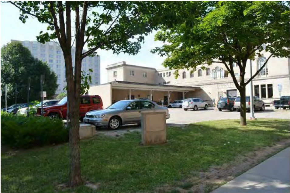
V11 - Existing site & MMB from the Pinckney & Doty intersection
