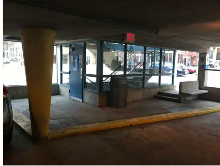
Existing Interior at West Corner of Garage
