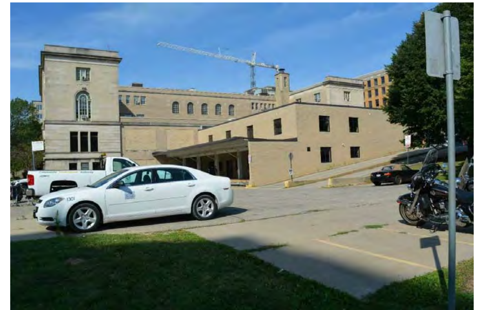
V6 - Existing site & MMB from Pinckney Street
