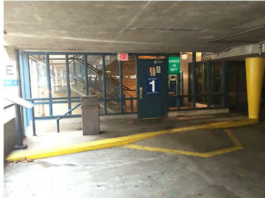
Existing Interior at North Corner of Garage
