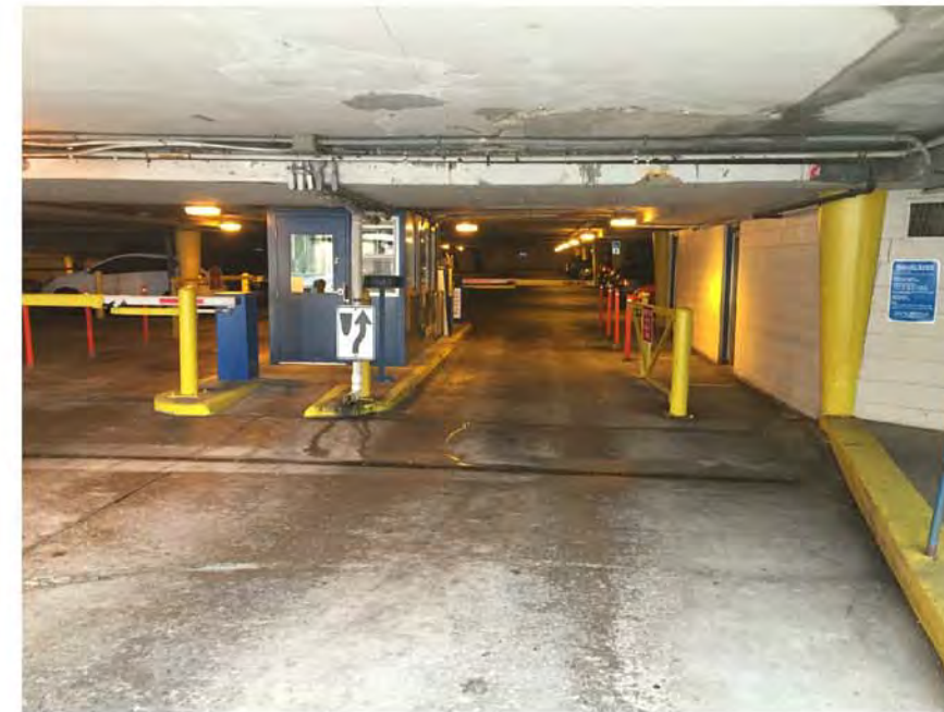
Existing Interior at Wilson Street Entrance
