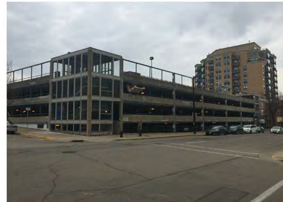
Existing Exterior from Pinckney & Wilson Intersection
