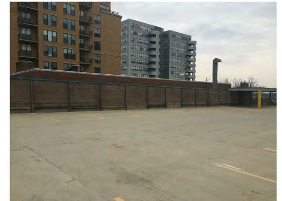
Existing Interior at Rooftop Looking East
