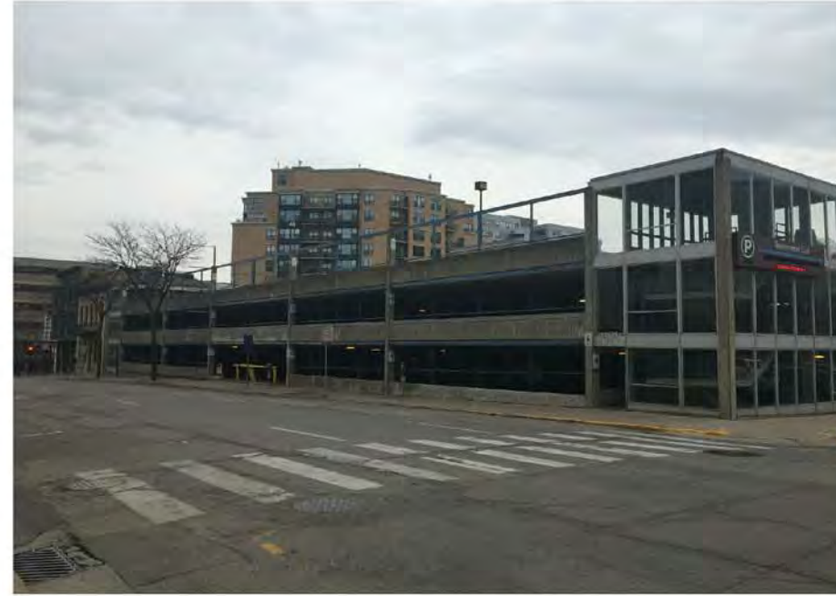
Existing Exterior Along Doty Street
