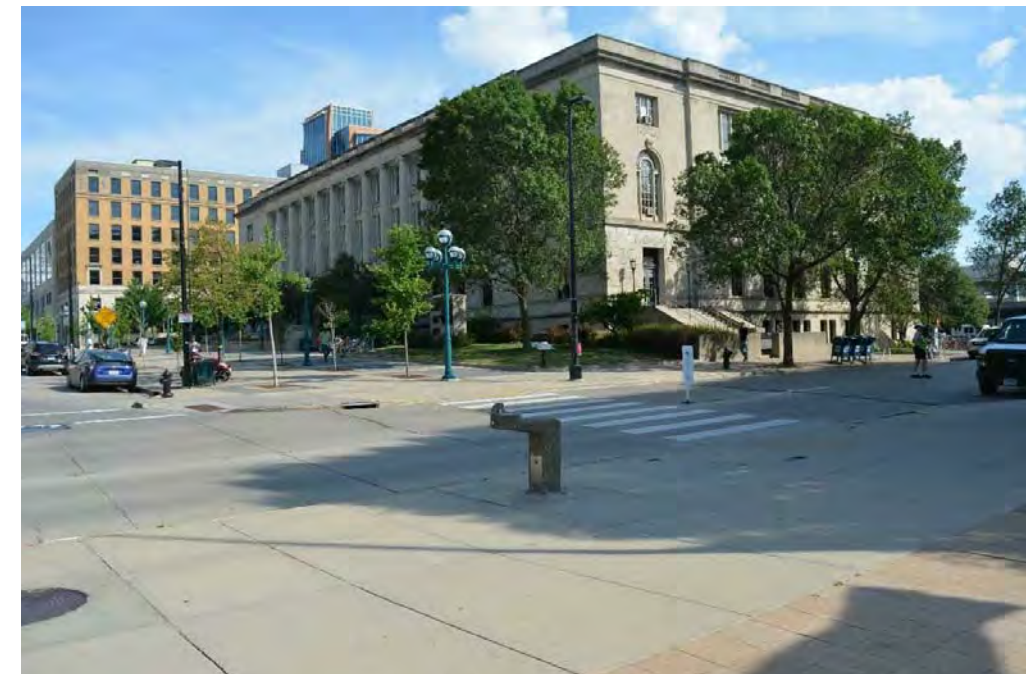
V1 - Madison Municipal Building from the Southwest
