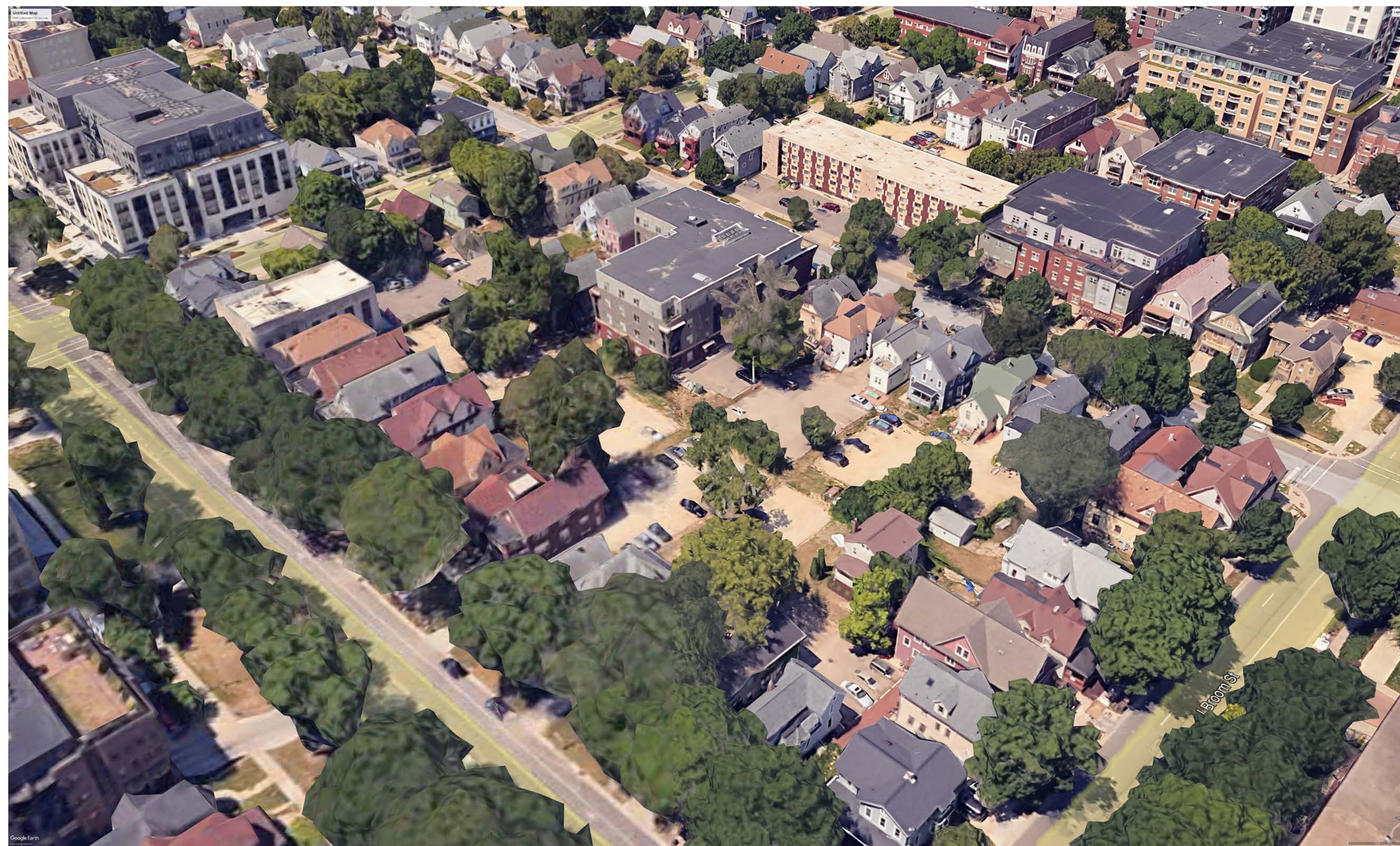
Aerial View - Washington Ave
