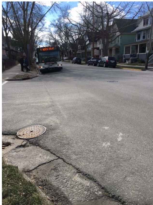
Image 5: Northbound Ingersoll looking west obstructed ped view far side
