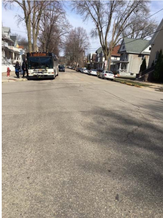
Image 14: Southbound Ingersoll looking east obstructed ped crossing far side
