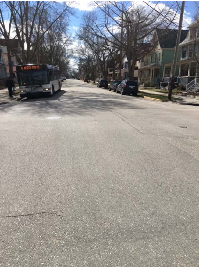
Image 6: Northbound Ingersoll looking west obstructed ped view crossing far side
