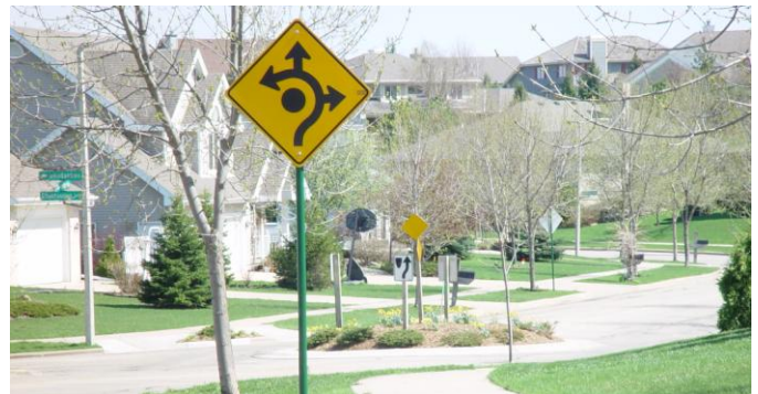
Permanent installation of a traffic circle at New Washburn way and Dandaneau Trail
