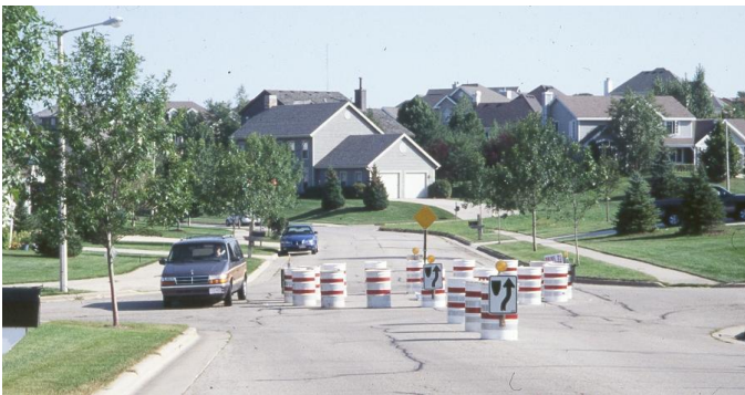
Temporary installation of a traffic circle at New Washburn way and Dandaneau Trail
