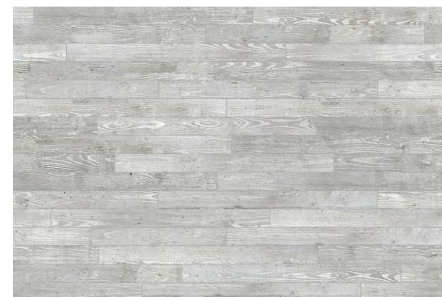
BOARD FORMED CONCRETE
