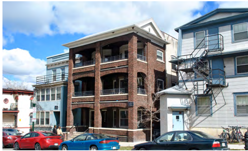
200 North Pinckney looking Northeast
