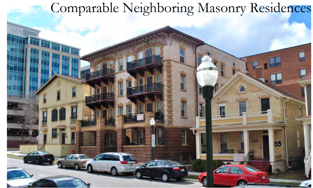
200 North Pinckney looking Southwest
