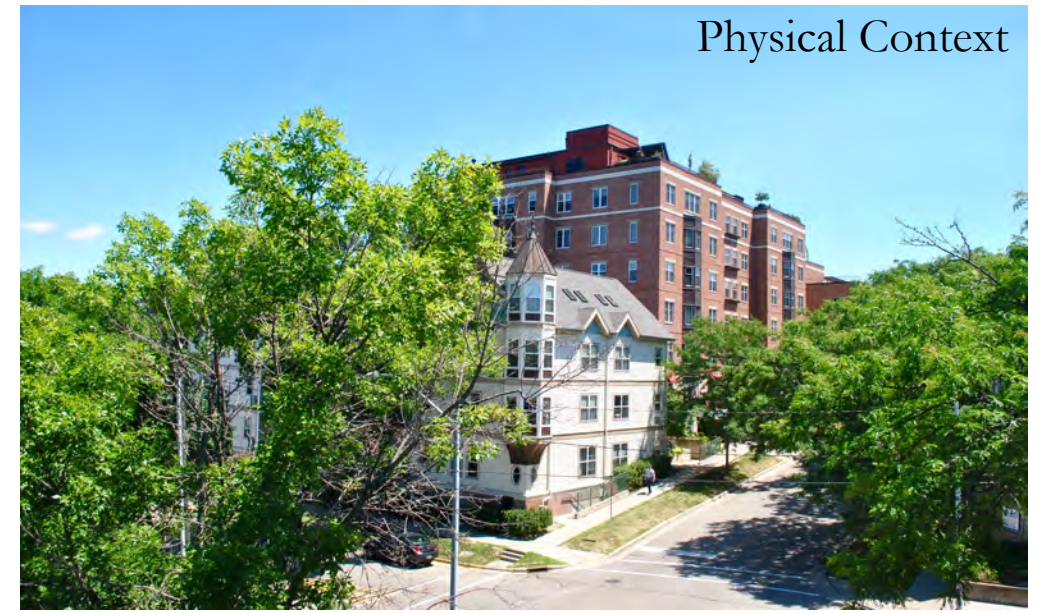
00 block of North Butler looking Northeast
