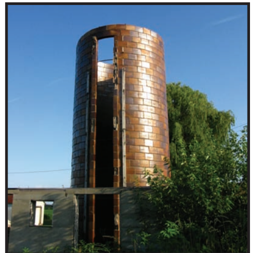
Glazed Tile Silo before deconstruction
