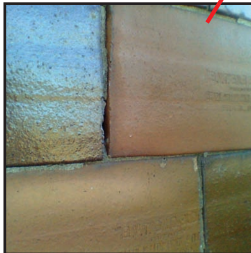
Closeup of Tiles
