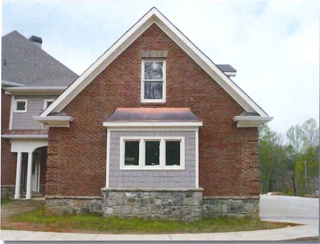
Photo 8 – Example of roof with eyebrow feature
