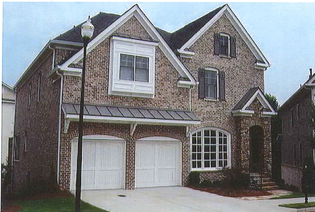
Photo 9 – Example of roof with eyebrow feature
