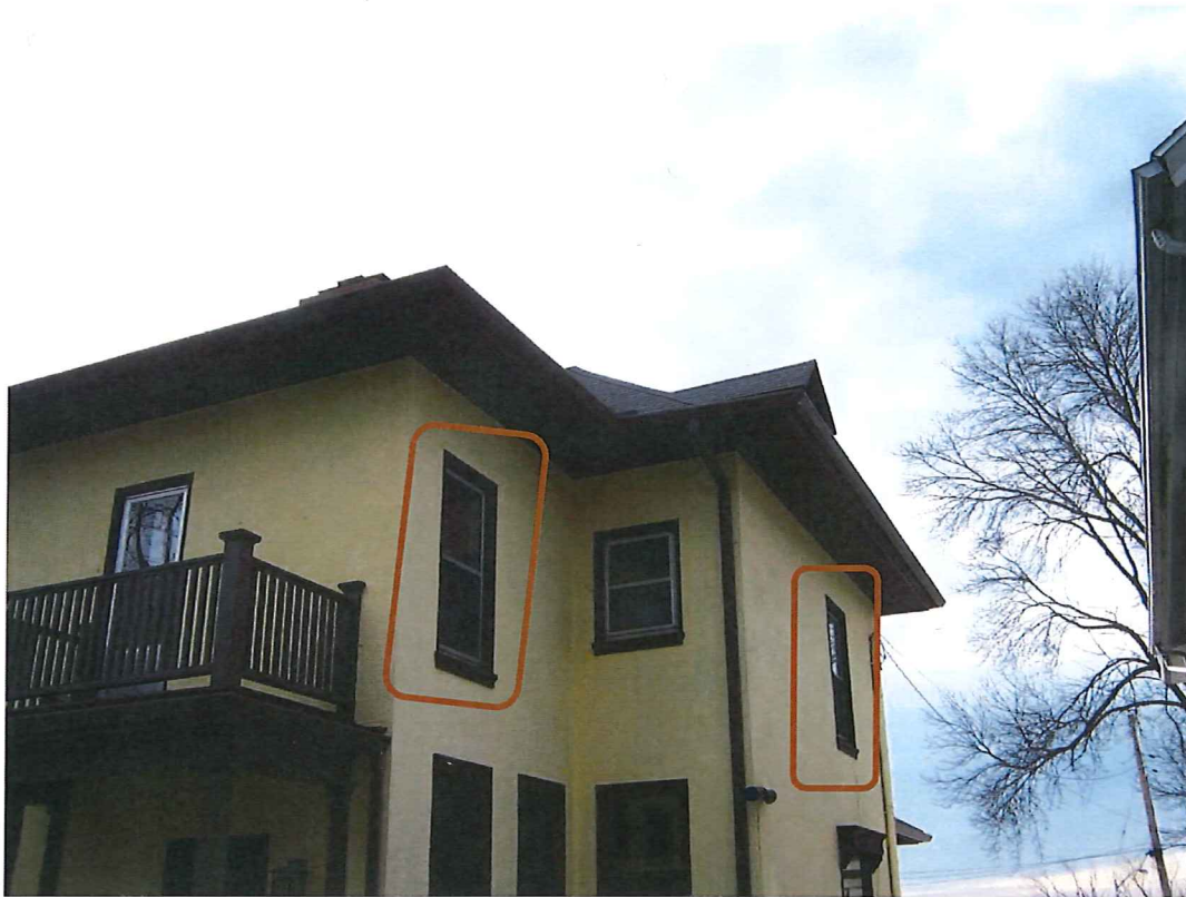
Photo 5 – 848 Spaight Street – 2 nd floor window replacement (left)
