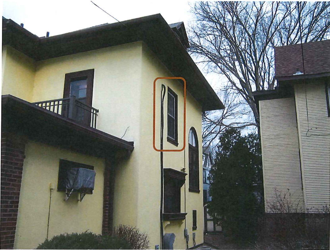
Photo 3 – 848 Spaight Street – 2 nd floor window replacement (right)
