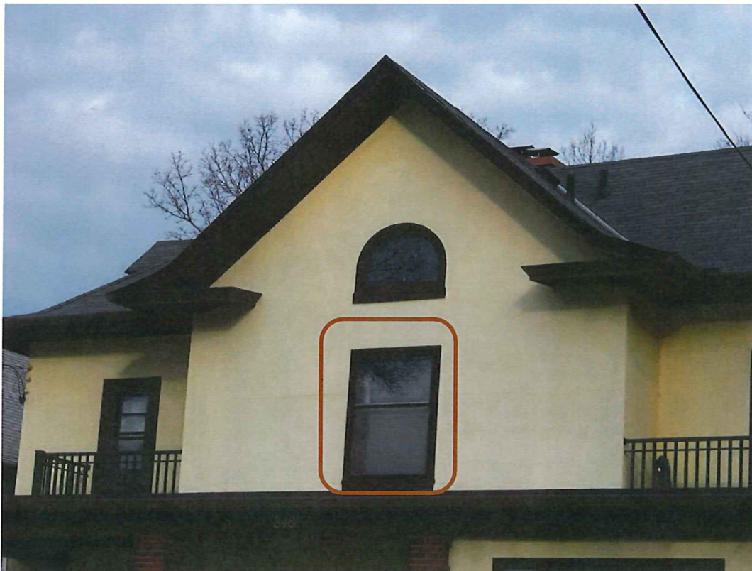
Photo 2 – 848 Spaight Street – 2 nd floor center window & center roof feature
