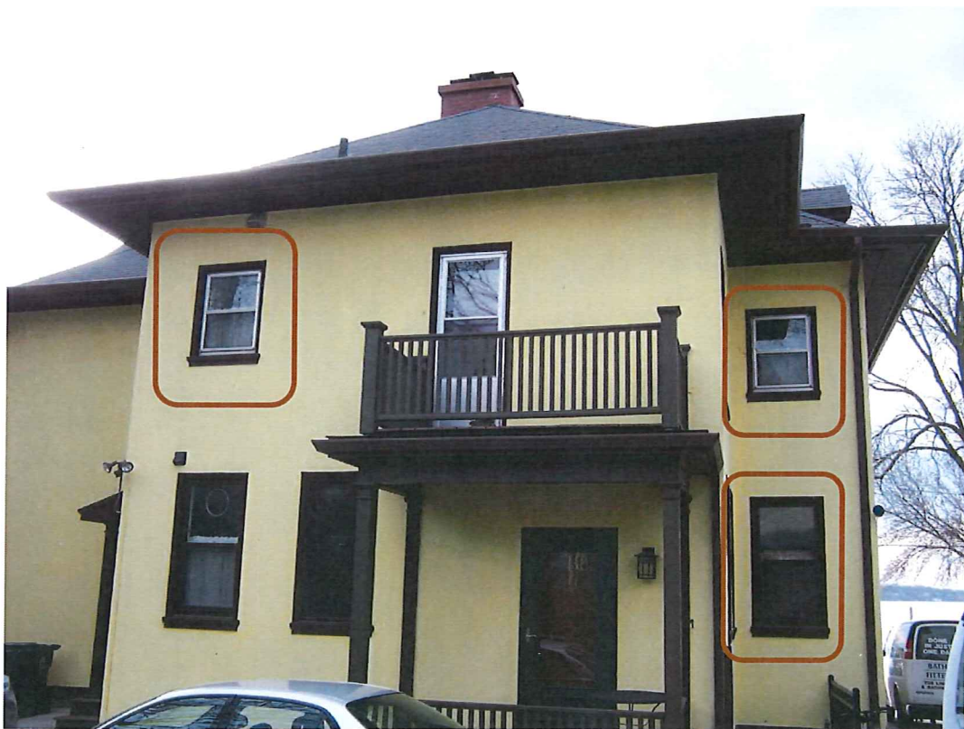
Photo 4 – 848 Spaight Street – window replacements (rear)
