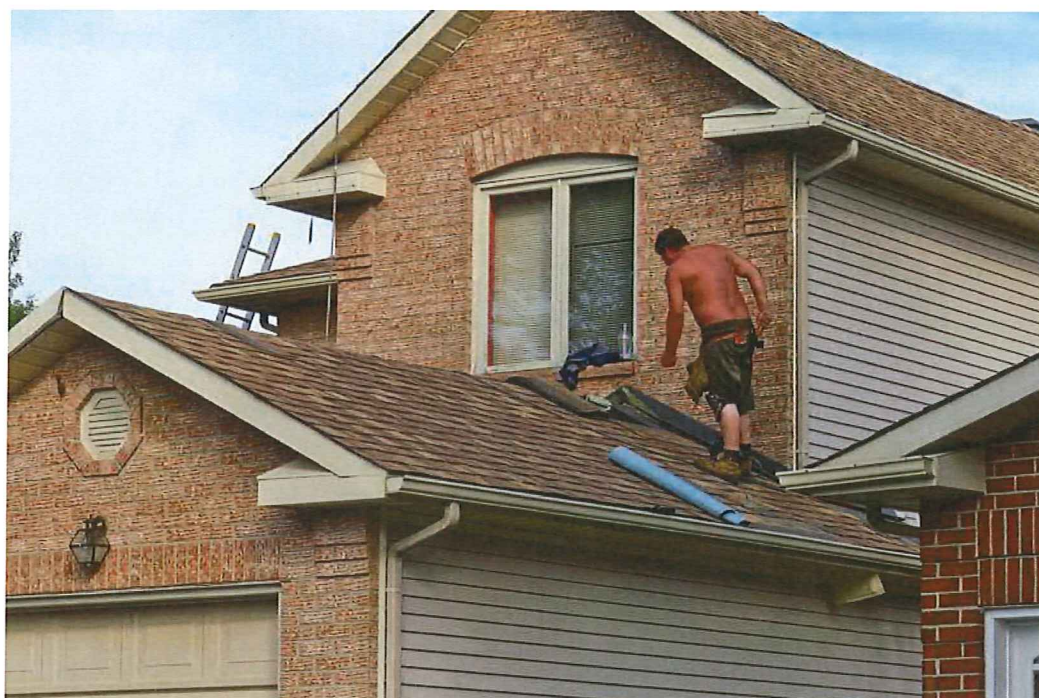
Photo 10 – Example of roof with eyebrow feature
