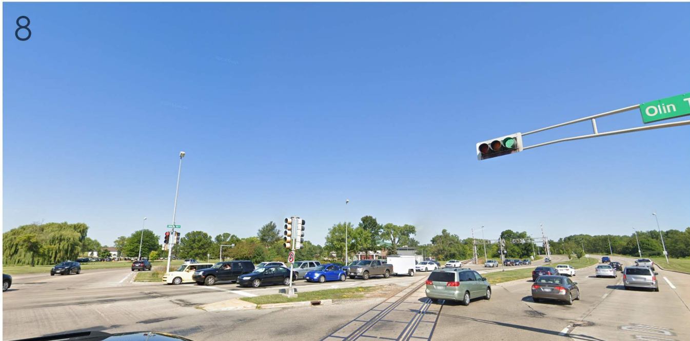
8: OLIN-TURNVILLE CT - FACING WEST
