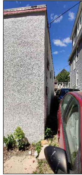
VIEW FROM REAR OF BUILDING LOOK TOWARDS W MIFFLIN
