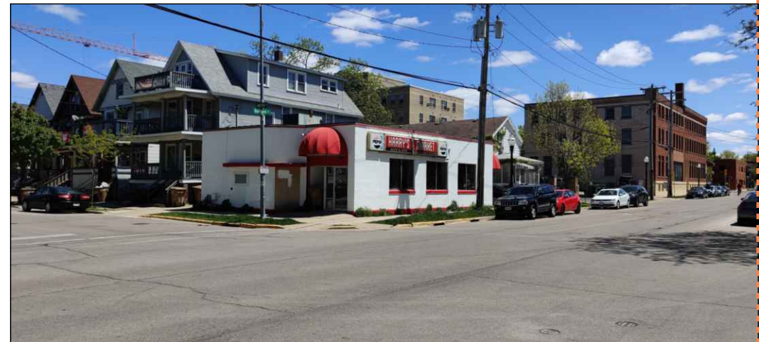
VIEW FROM BEDFORD & W MIFFLIN LOOKING AT MAIN ENTRY
