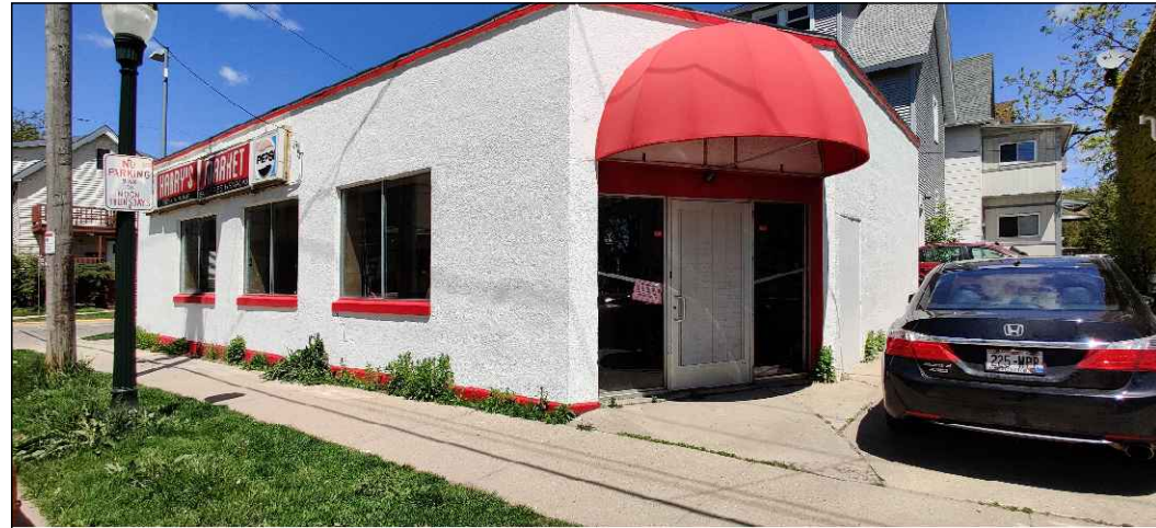
VIEW FROM BEDFORD LOOKING AT REAR ENTRY
