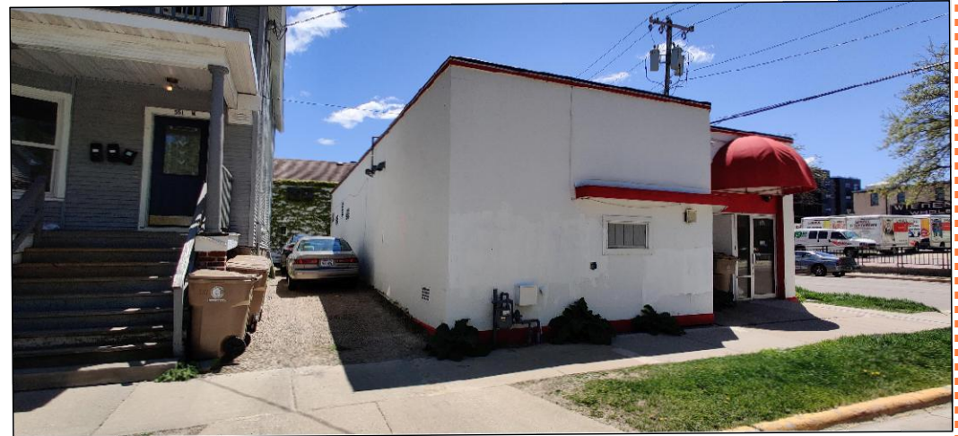
VIEW FROM W MIFFLIN LOOKING AT REAR OF BUILDING & MAIN ENTRY
