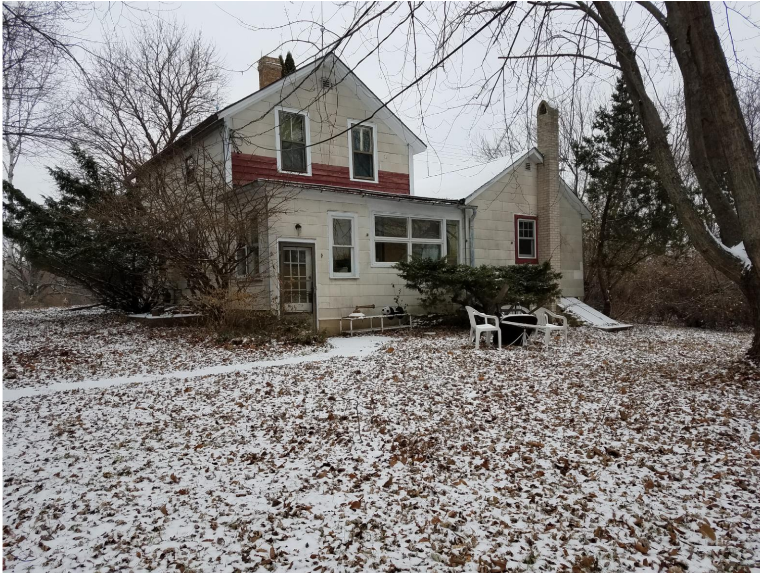
Existing house on site to be demolished
