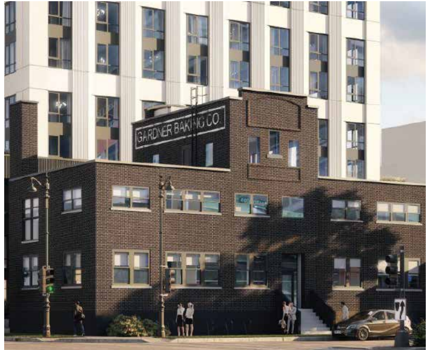
2ct. Repaint 1920's Historical Wall Signage Back to Original White Condition
