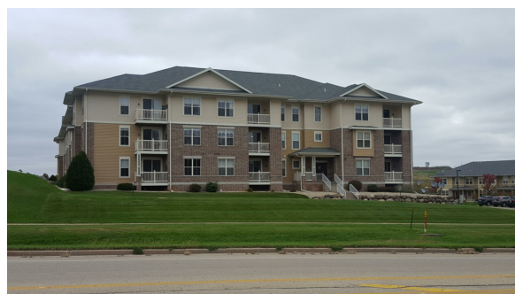
48 Unit Bldg from Nelson Rd. to N.
