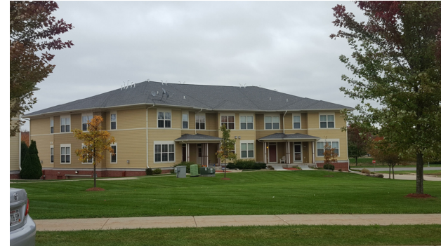
Rear of 9 Unit Building
