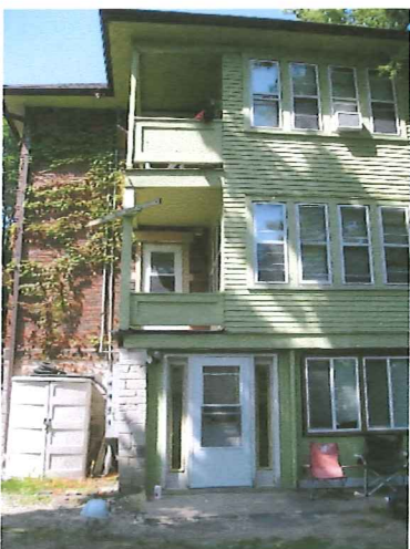
South Side, Subject Bldg
