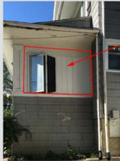
SIDE OF PORCH
