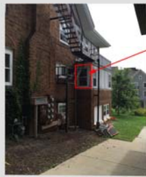
SIDE VIEW OF PORCH
