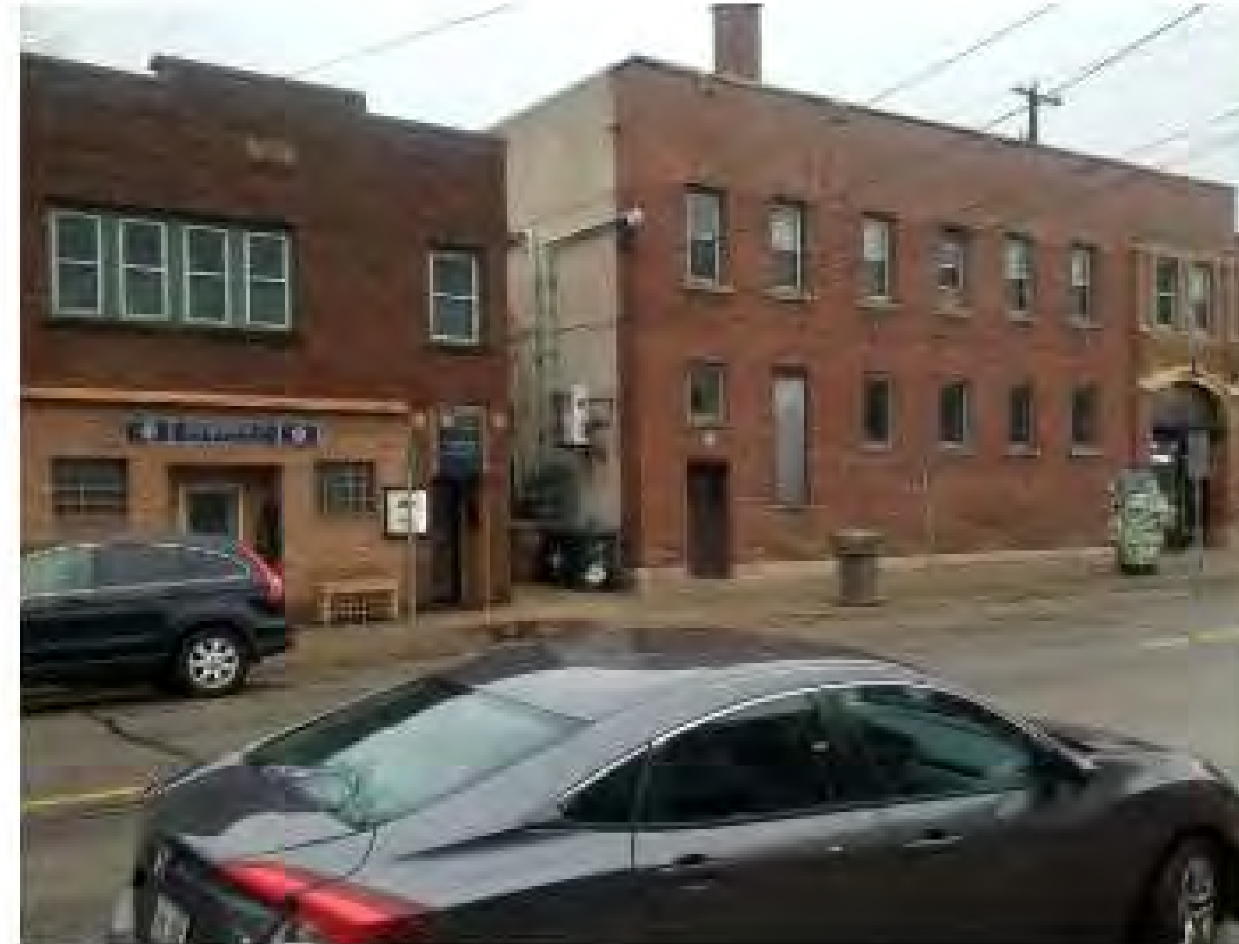
408 SOUTH BALDWIN ST.
