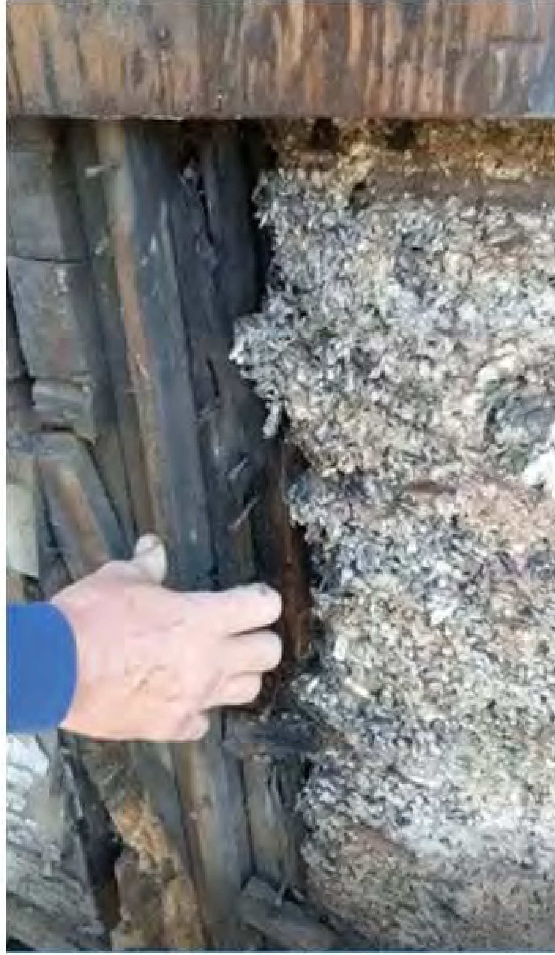
EXTERIOR WALL INVESTIGATION
