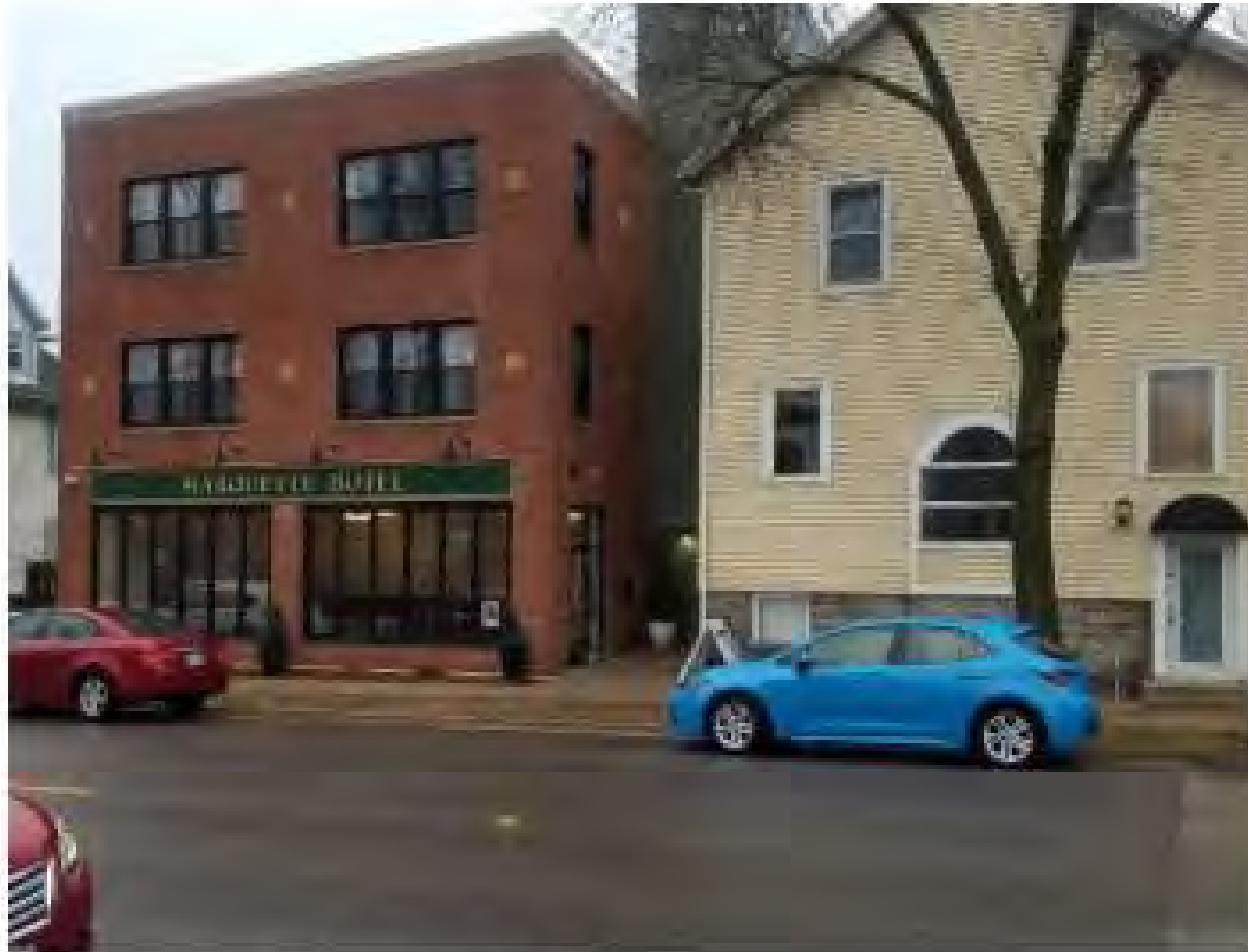
414 SOUTH BALDWIN ST.
