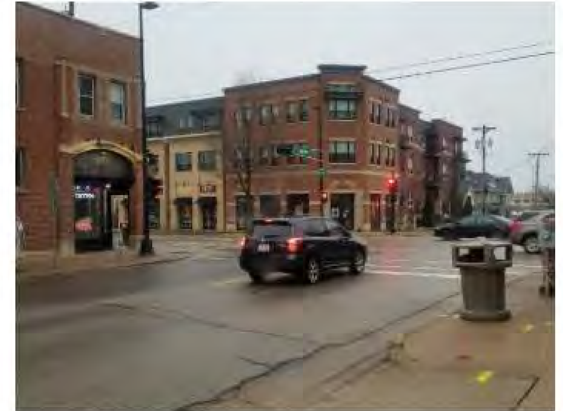
320 SOUTH BALDWIN ST.
