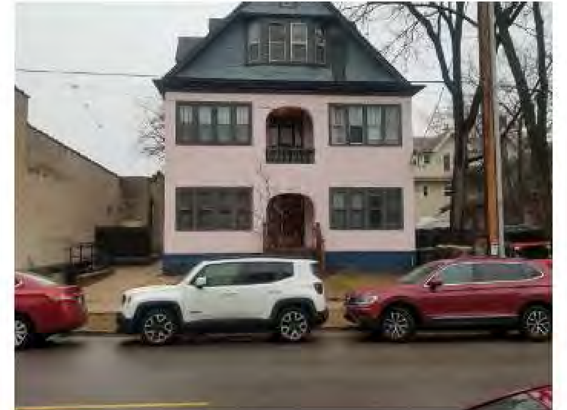
413 SOUTH BALDWIN ST.
