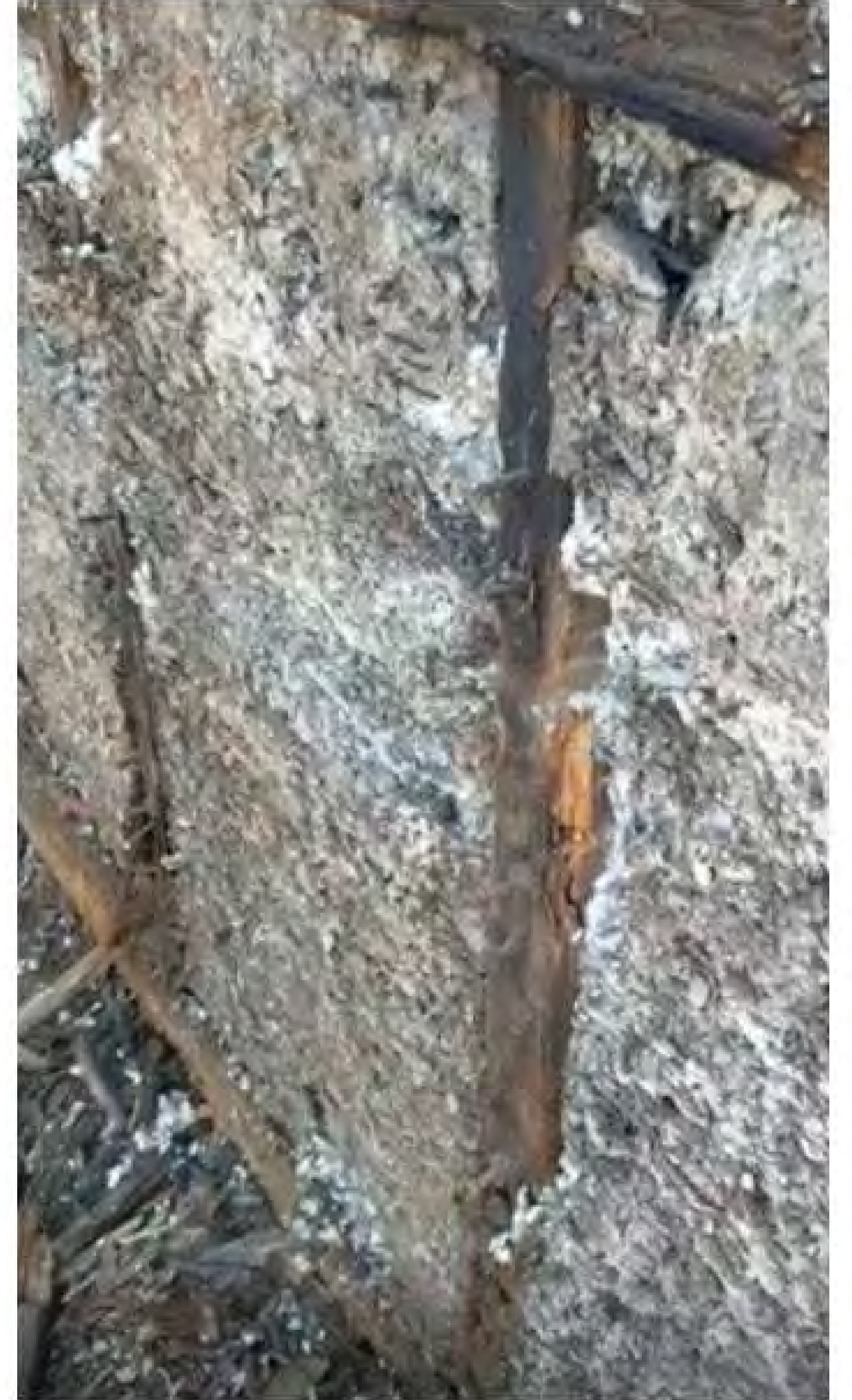
EXTERIOR WALL INVESTIGATION
