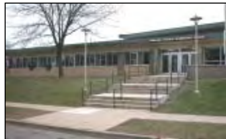
The entrance of Lincoln Elementary School is off Sequoia Trail. Aesthetic improvements, such as new plantings, in front of the building would make it more appealing.
