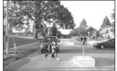
Installation of traffic islands on Cypress Way has increased pedestrian safety.
