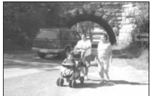
Access to Quann Park from the Bram's Addition Neighborhood is unsafe since pedestrians must walk through a narrow railroad viaduct.
