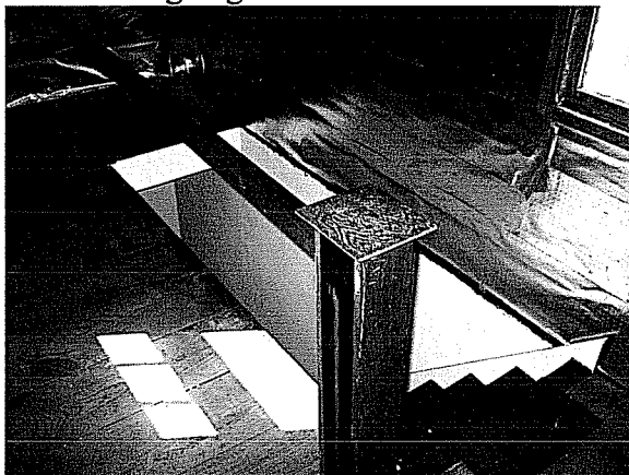
Stairwell out of code to second bedroom
