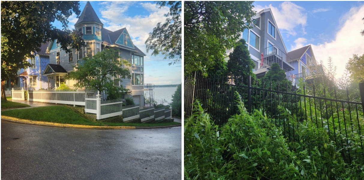
Figure 2. Example of an approved addition including casement windows and sliding doors at 1101 Rutledge St.
