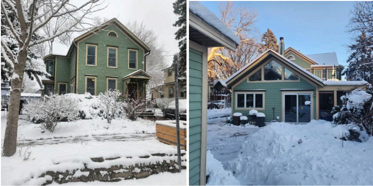
Figure 1. Example of 912 Spaight Street with an approved rear addition containing casement windows and sliding doors.
