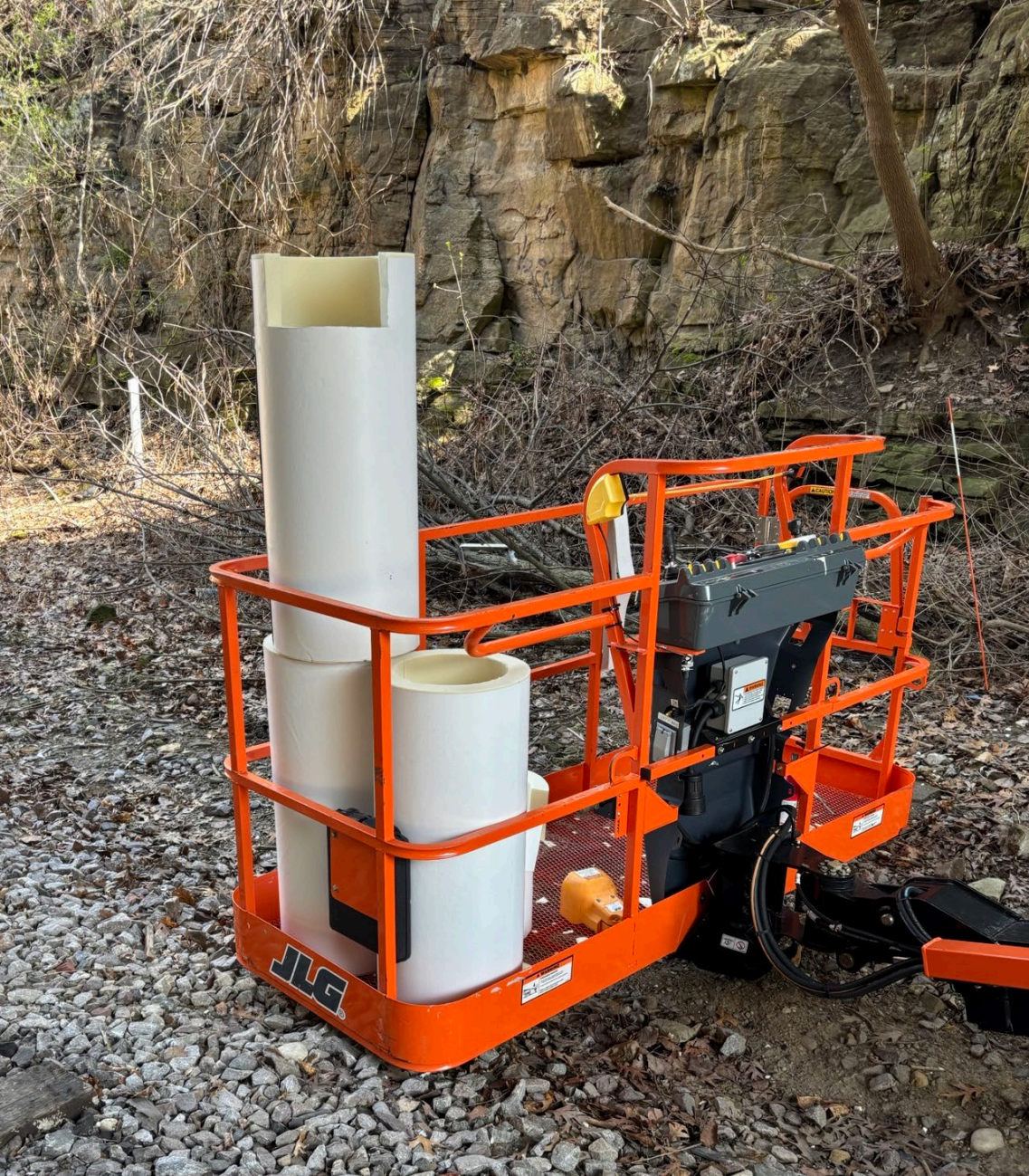
Photos: Insulation / Jacket Prep (Left) and Partial Application (Right)
