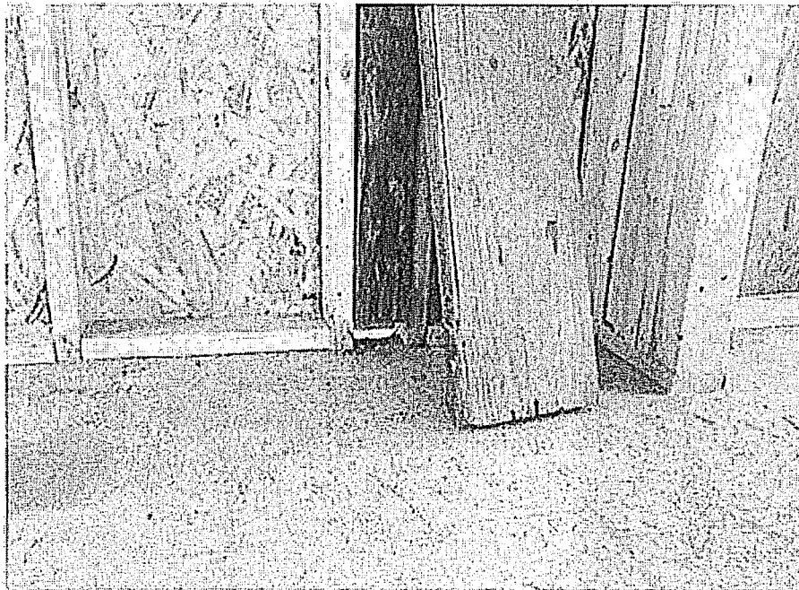
Image 40: Wall framing at perimeter.
