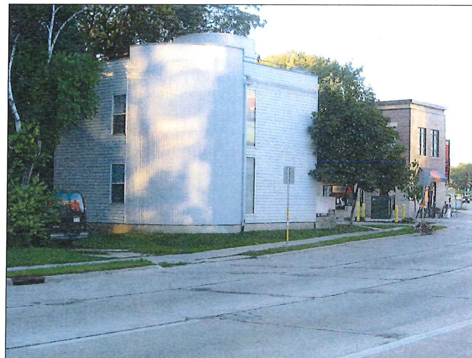
LOOKING SOUTH DOWN PARK STREET
