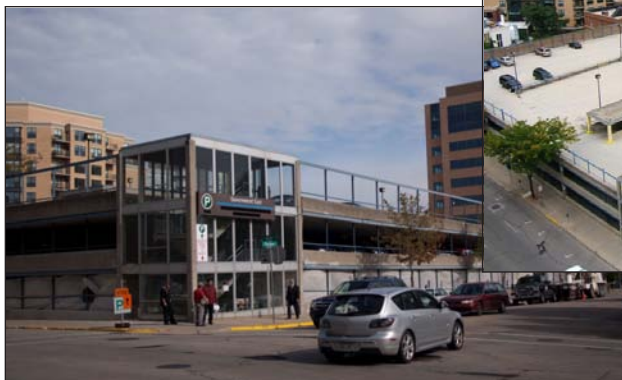
Government East Parking Garage, 2012
