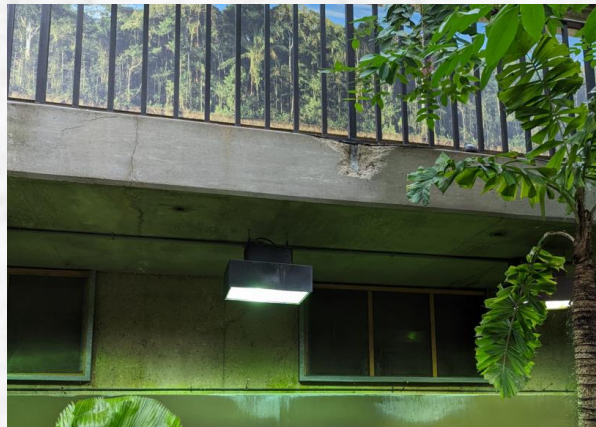
Cracks and spalling at elevated walkway
