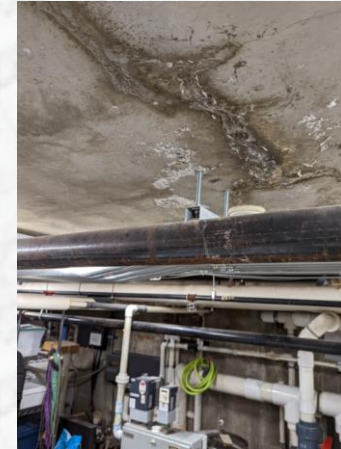
Water leaks from planter box and/or upper waterfall over plumbing mechanical equip.
