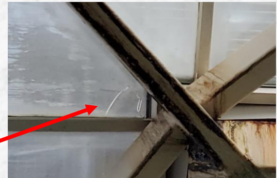
Water leaks from planter box and/or upper waterfall over plumbing mechanical equip.
