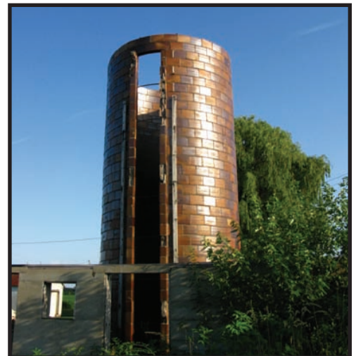
Glazed Tile Silo before deconstruction
