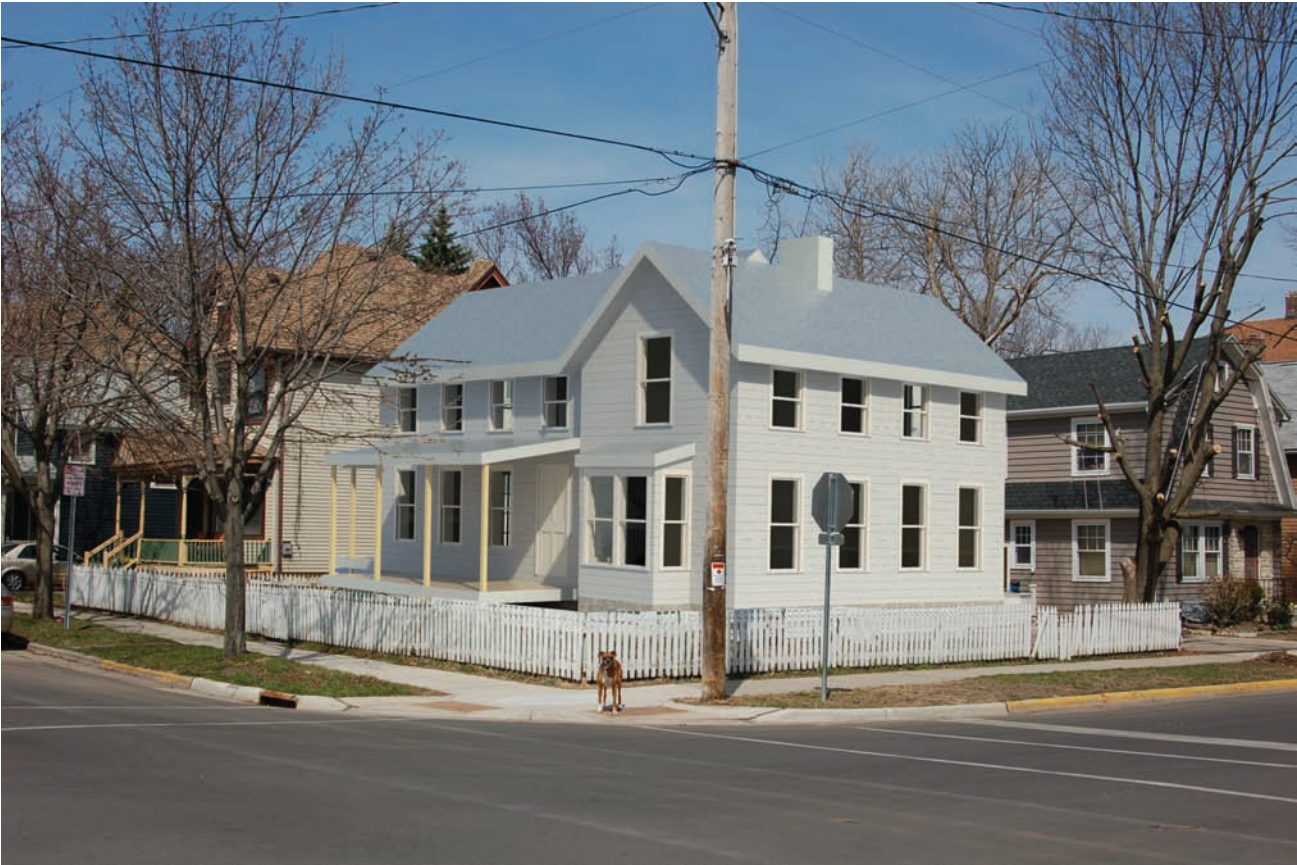
VIEW FROM INTERSECTION
