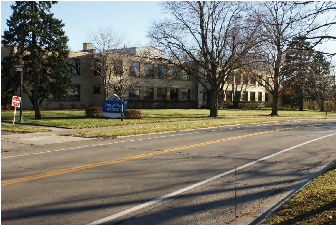
Filene House West Elevation, Photo from Northwest 11.25.22.
