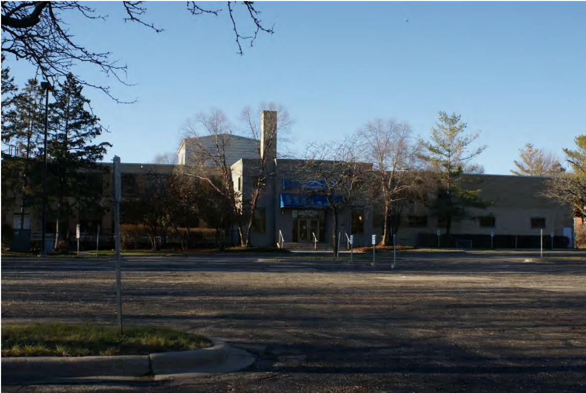
Filene House East Elevation. Photo from East 11.25.22.
