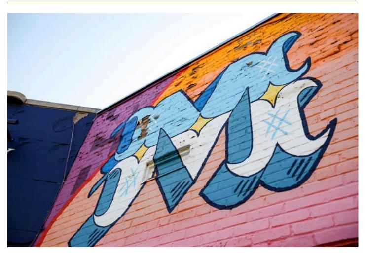
The "M" in the "MADISON" mural has the most damage, with many of the original bricks peeking out and some of the paint flaking off due to brick damage.
