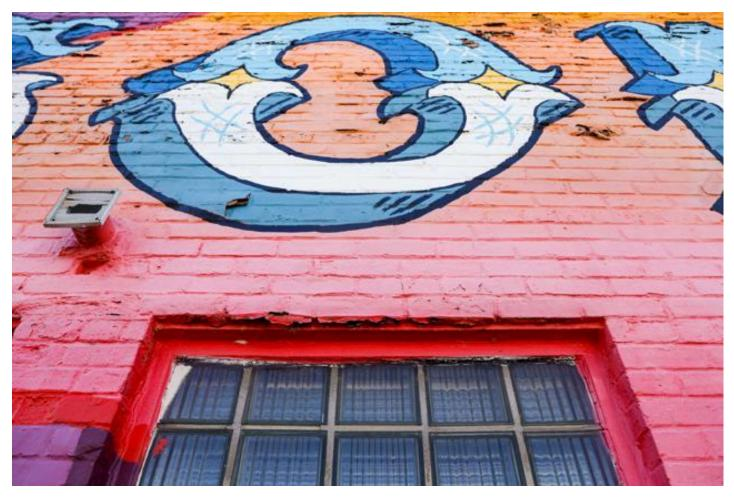
The mural shows some of the structural damage from the deteriorating brick below. The owners of Lauer Realty are replacing the brick and have no plans to replace the mural.
