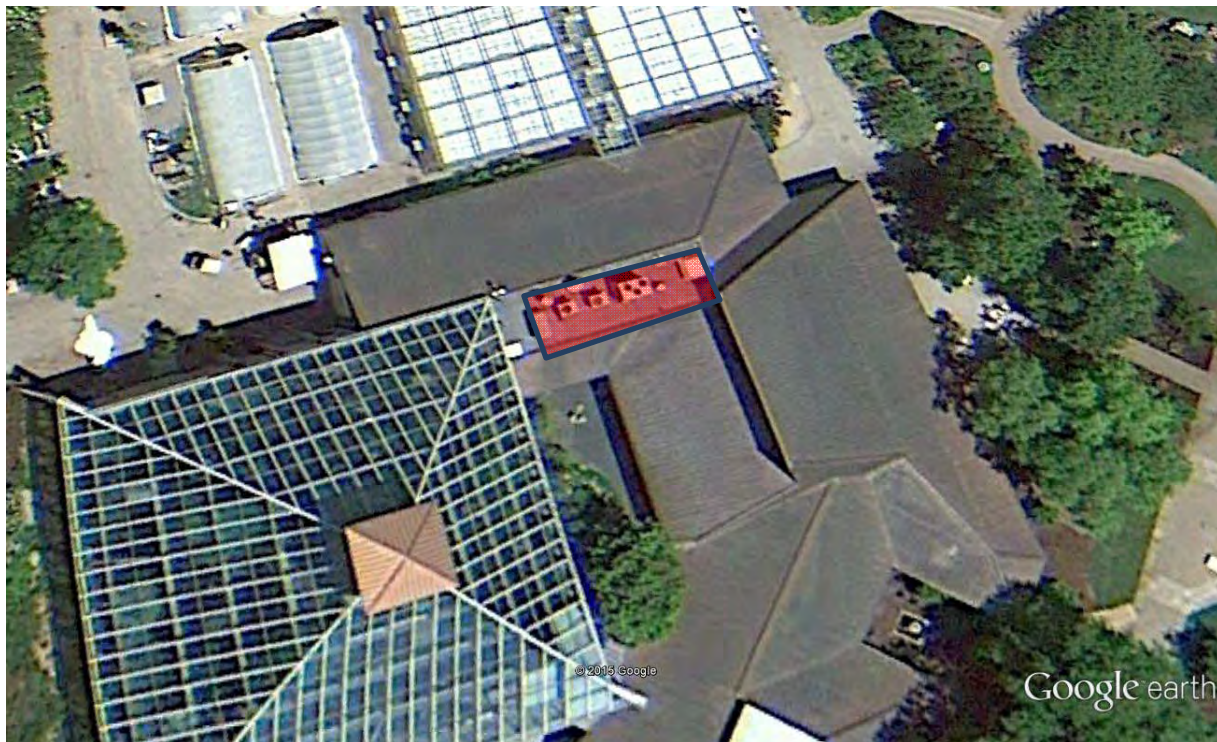
Figure 1 – Aerial photo provided by Google Earth showing Olbrich Garden roof area available for possible solar hot water collector sites (highlighted in red)
