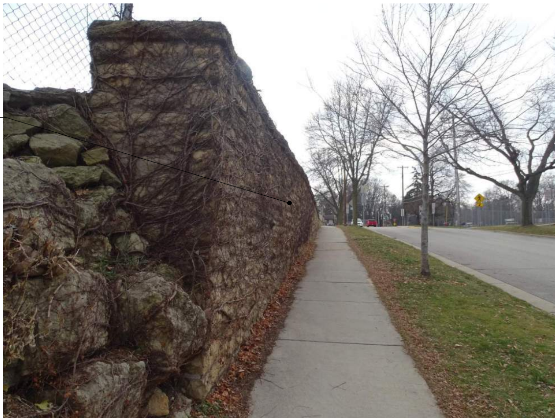
VIEW AT VAN HISE AND HIGHLAND LOOKING SOUTH
