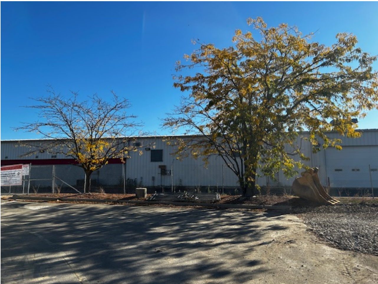
Exterior – SE Elevation; 10-7-2024
