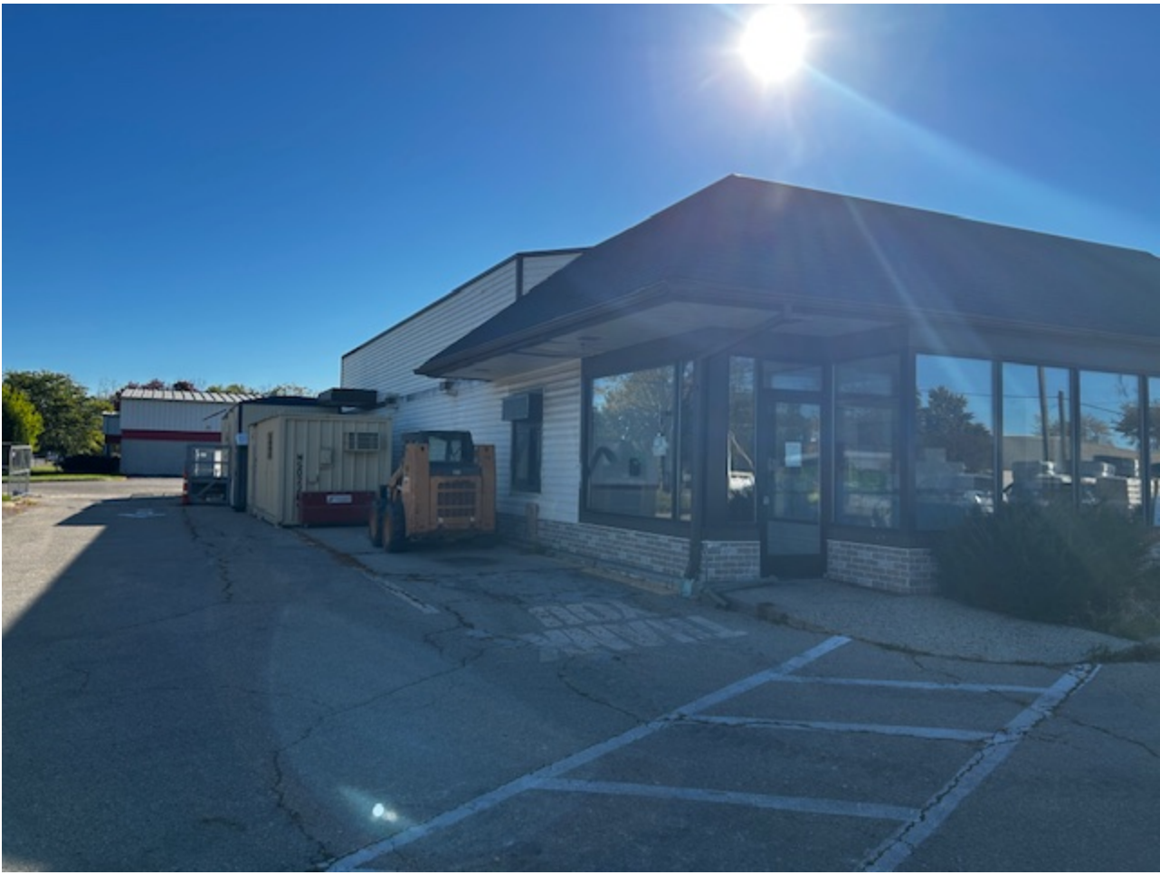
Exterior – South Elevation; 10-7-2024
