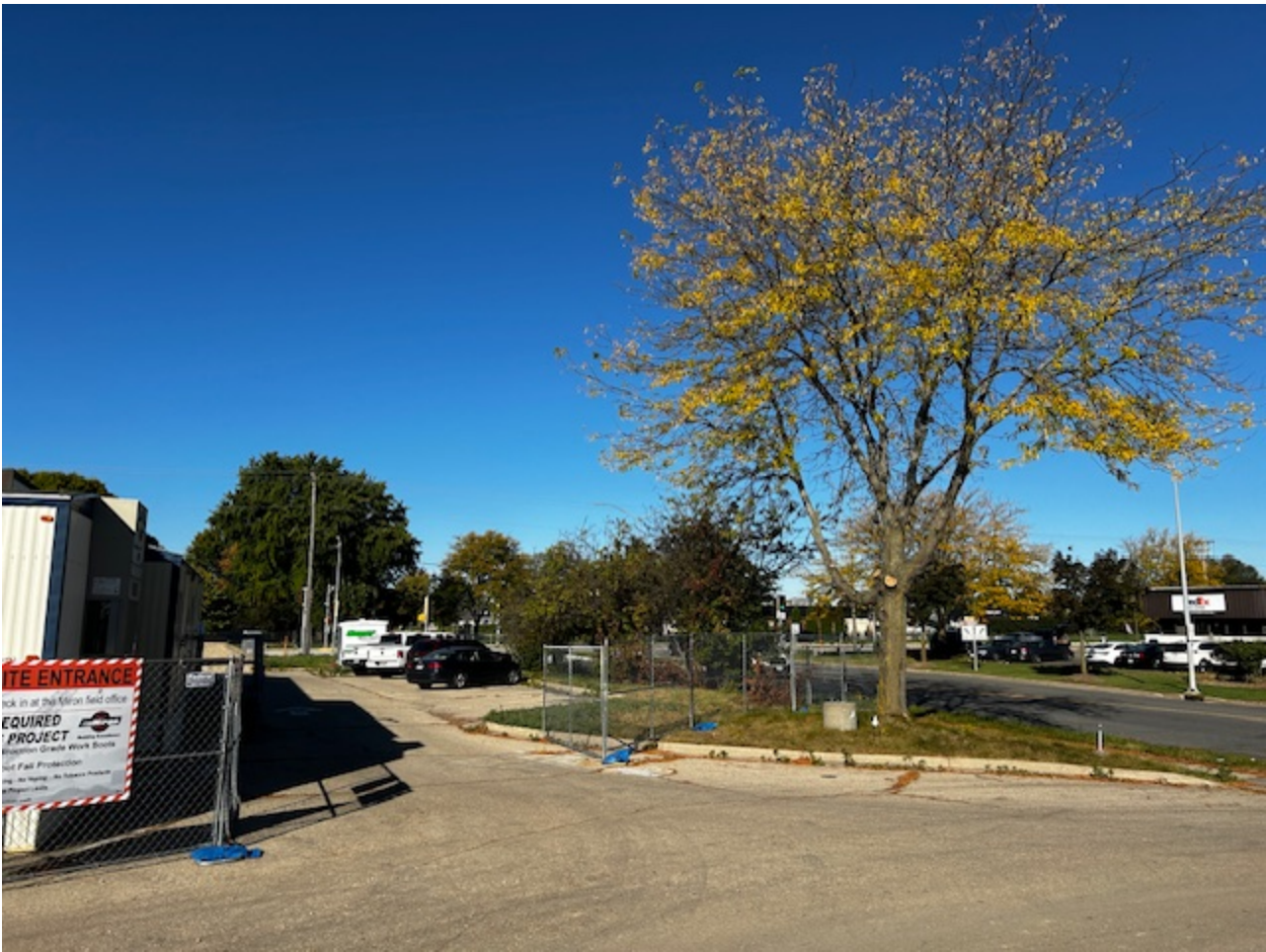
Exterior East Property Line; 10-7-2024
