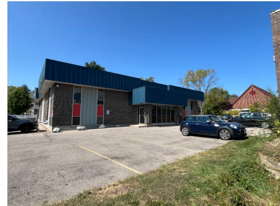
VIEW OF EAST SIDE OF BUILDING
