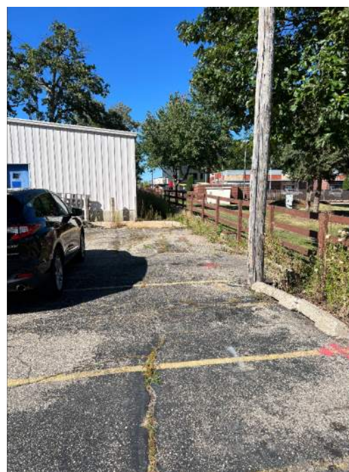
EXTERIOR EAST EDGE OF LOT
