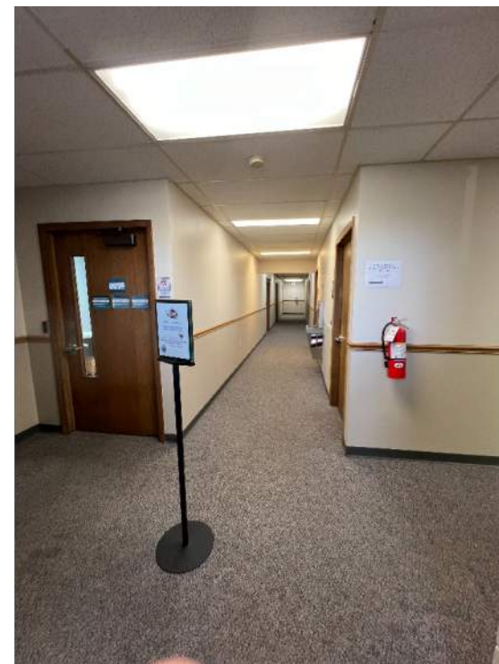
LOWER LEVEL HALL TO OFFICES
