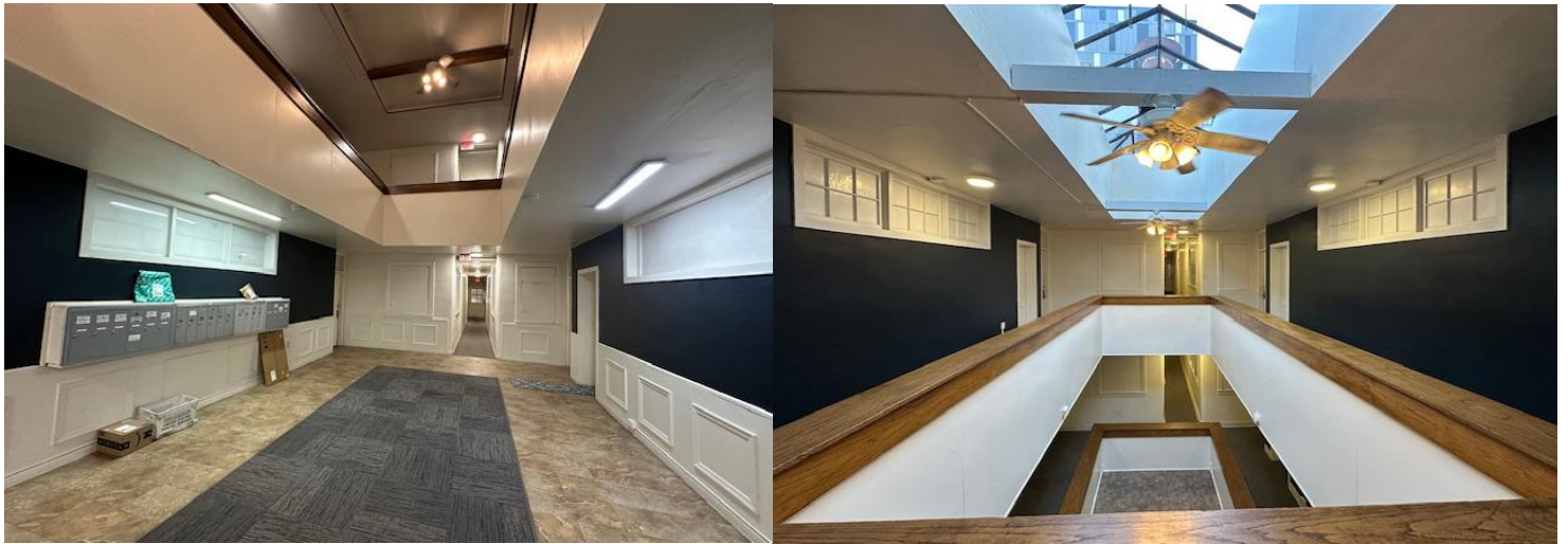
Non-separated floor between apartment unit levels.
