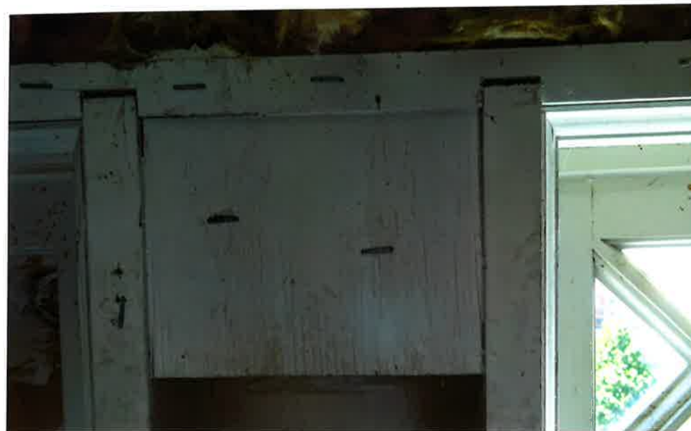
3rd FLOOR WINDOW PHOTO SURVEY- FRONT
