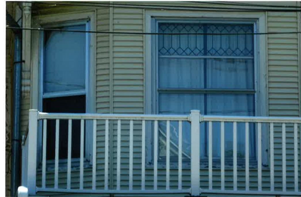
2nd FLOOR WINDOW PHOTO SURVEY - TO BE RETAINED
