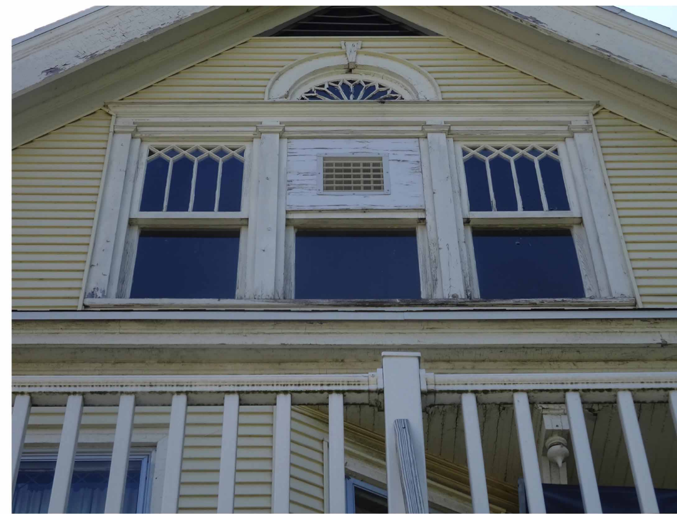
3RD FLOOR WINDOW GROUP
