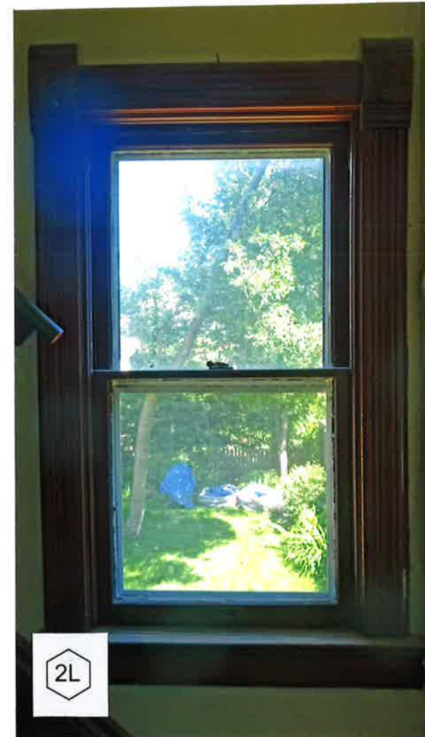
2nd FLOOR WINDOW PHOTO SURVEY - TO BE RETAINED
