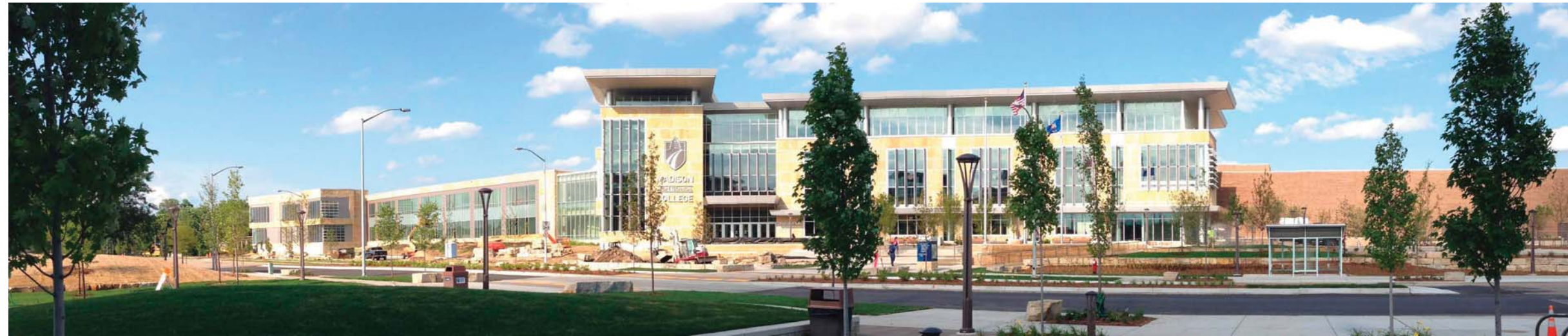
C1: VIEW LOOKING EAST FROM WRIGHT STREET TO THE TRAUX BUILDING/MITBY THEATER/REDSTEN GYMNASIUM
