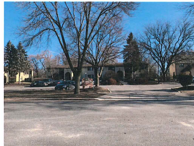
709-11 McCormick Street to East – Mid-Block 1
