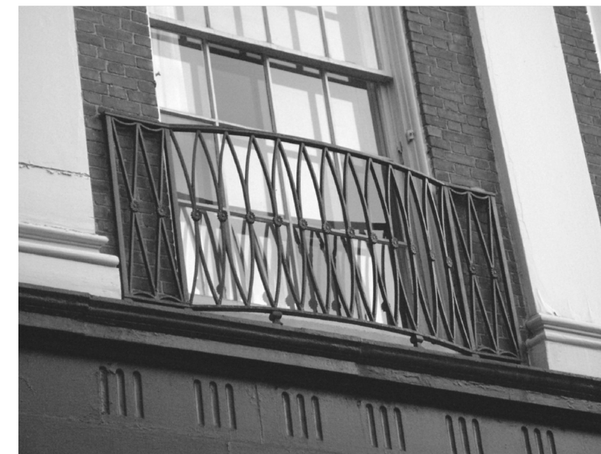
2 Painted Metal Railing Reference Image SCALE: N.T.S.
