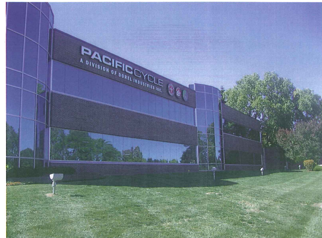
VIEW LOOKING SOUTH – BELTLINE SIDE
