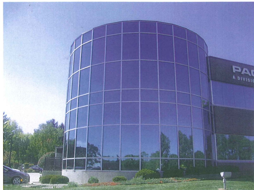
VIEW LOOKING SOUTH – BELTLINE SIDE
