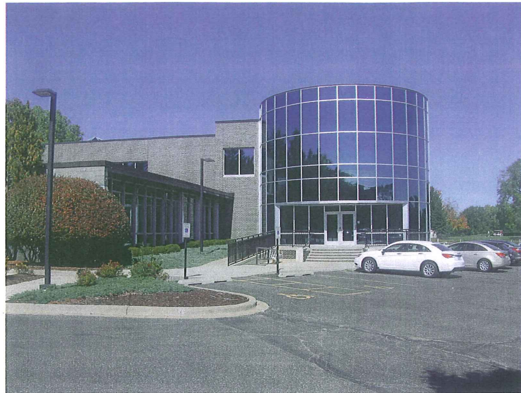
VIEW LOOKING NORTH – MAIN ENTRANCE
