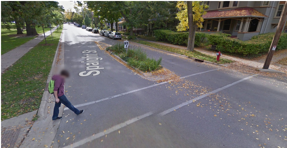
Figure 7. Pedestrian refuge island example (Spaight St at Orton Park).
