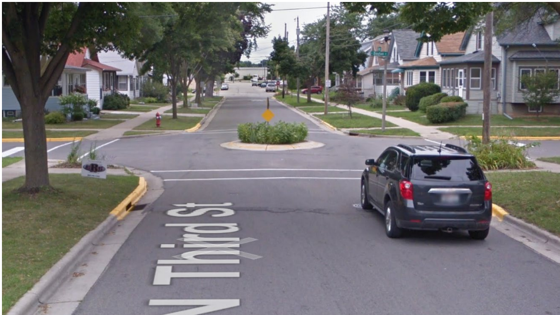
Figure 5. Traffic circle example (N Third St & E Dayton St).
