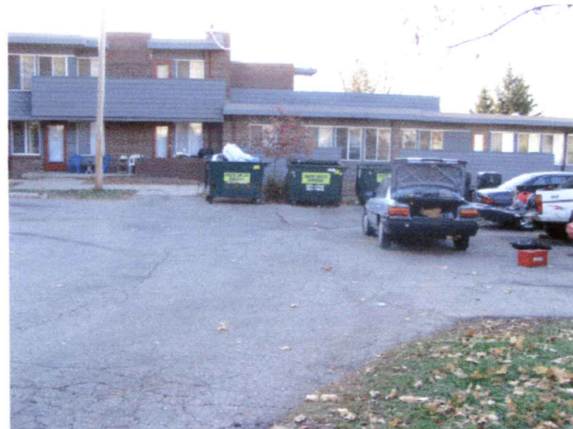
1850 Beld Street Cracked drive, unsecured trash containers October 25, 2003
