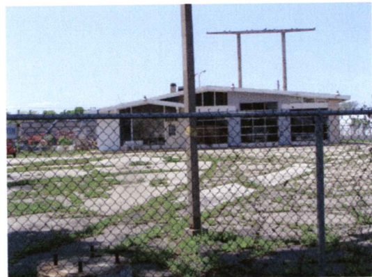
1010 Ann Street Abandoned sign posts, blighted parking areas October 25, 2003
