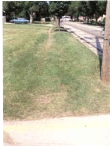
Badger Road Missing Sidewalk July 7, 2005
