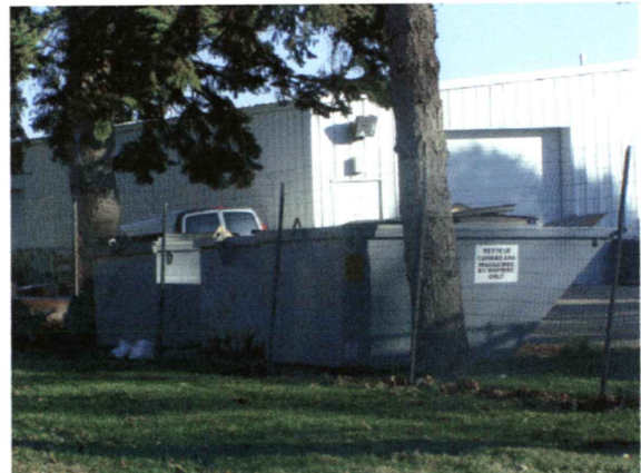
1114 Ann Street Unscreened trash container October 25, 2003
