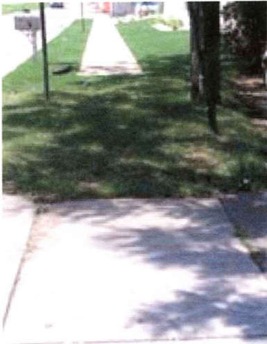
Perry Street Missing Sidewalk July 7, 2005
