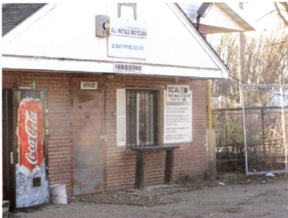
1818 South Park Street Deteriorated door October 25, 2003
