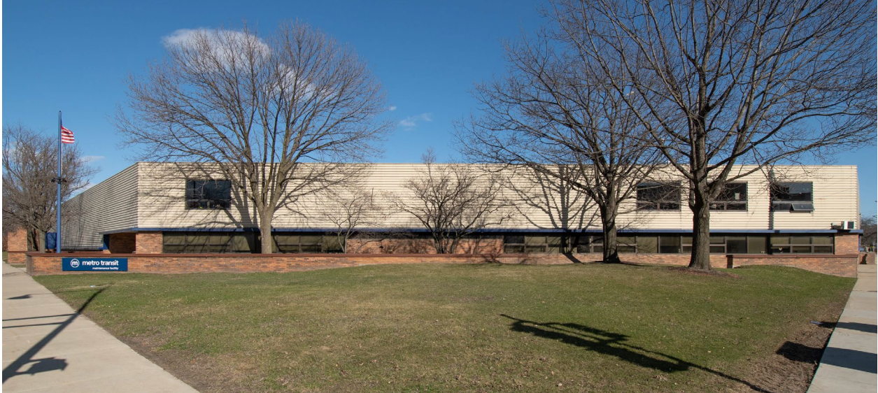
Image of the Metro Facility showing triangular green space at corner of Ingersoll and East Washington. Note low brick wall that creates inner paved area shown in image below. City of Madison photo.
