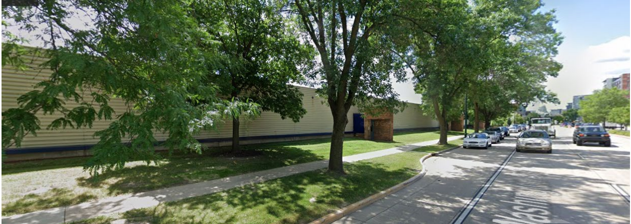
Google street view image of north building wall along East Washington.
