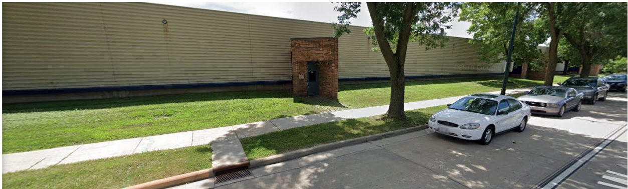
Google street view image of north building wall along East Washington.
