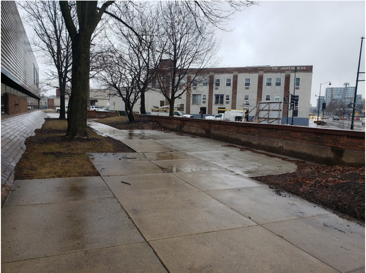
Metro Facility near corner of Ingersoll and East Washington showing the area inside the brick wall at the triangular green space. City of Madison photo.
