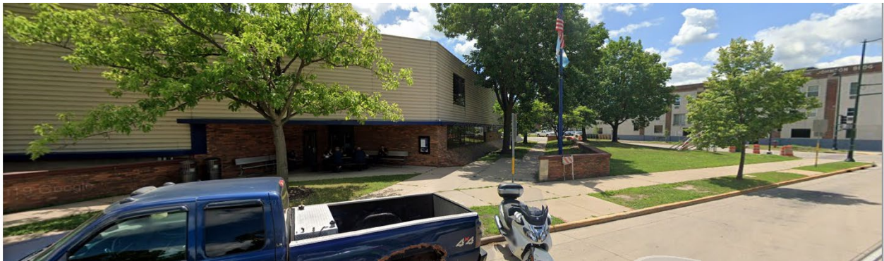
Google street view image of Metro Facility showing staff entrance and triangular green space at corner of Ingersoll and East Washington.
