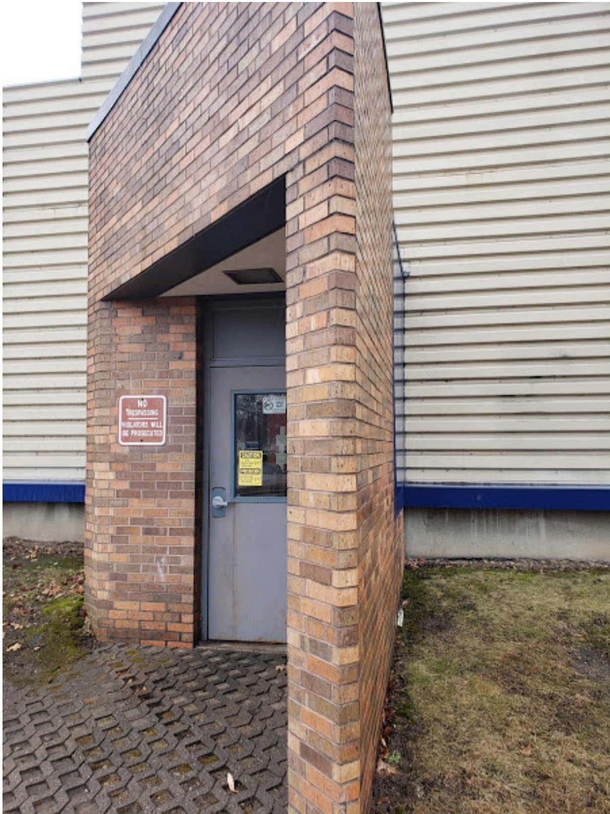
Egress portals project from the north providing the only indication of human scale. The portals have an angled expression and are clad in brick and blue metal panel which contrasts the horizontal siding used for the main body of the building.
