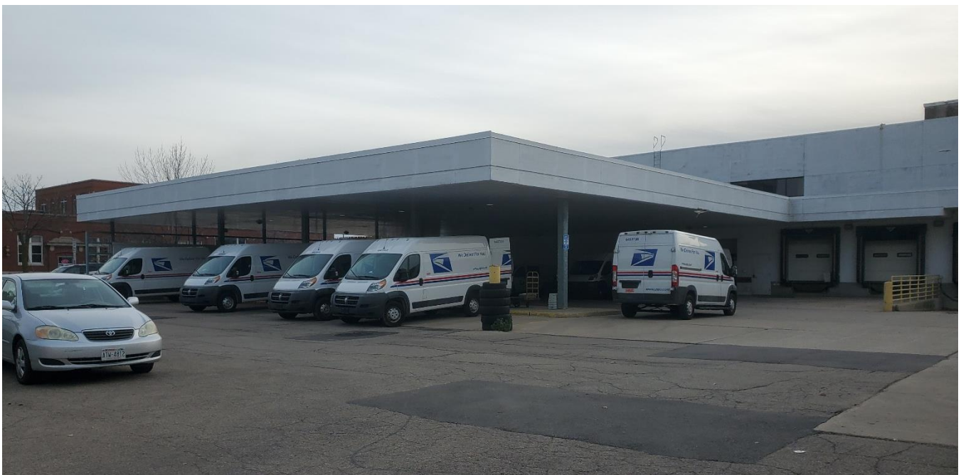
702 East Washington Avenue Vehicle canopy on southeast portion of parcel
