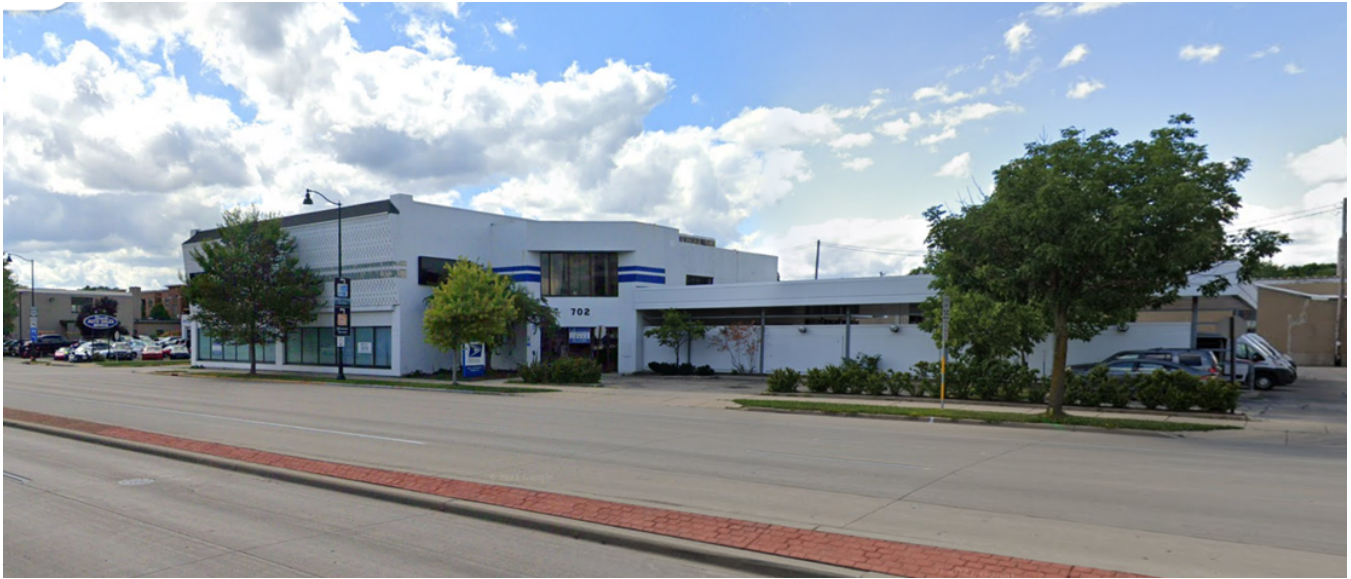
702 East Washington Avenue Looking northwest down East Washington Avenue
